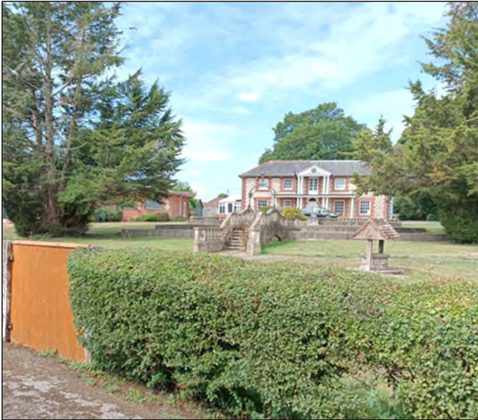
Photo 1: Main Former House Padnell Grange, facing west
