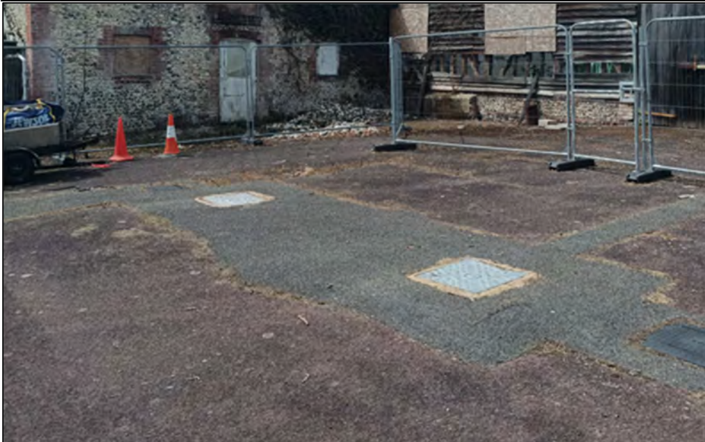
Photo 8: Drainage observed onsite.
