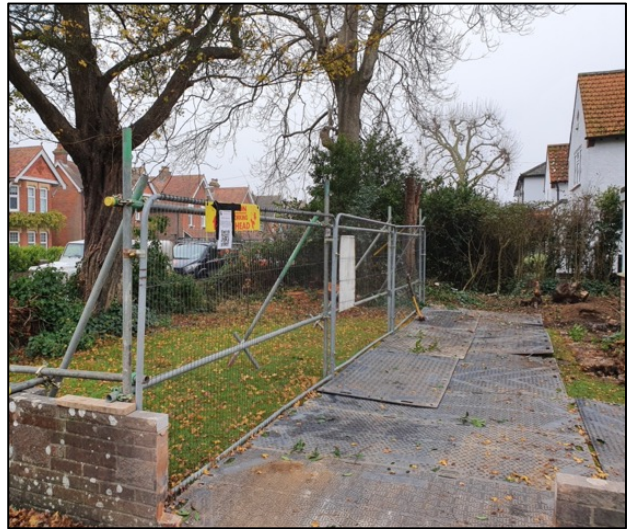
GP2: Tree protection barriers & trackmat ground protection
