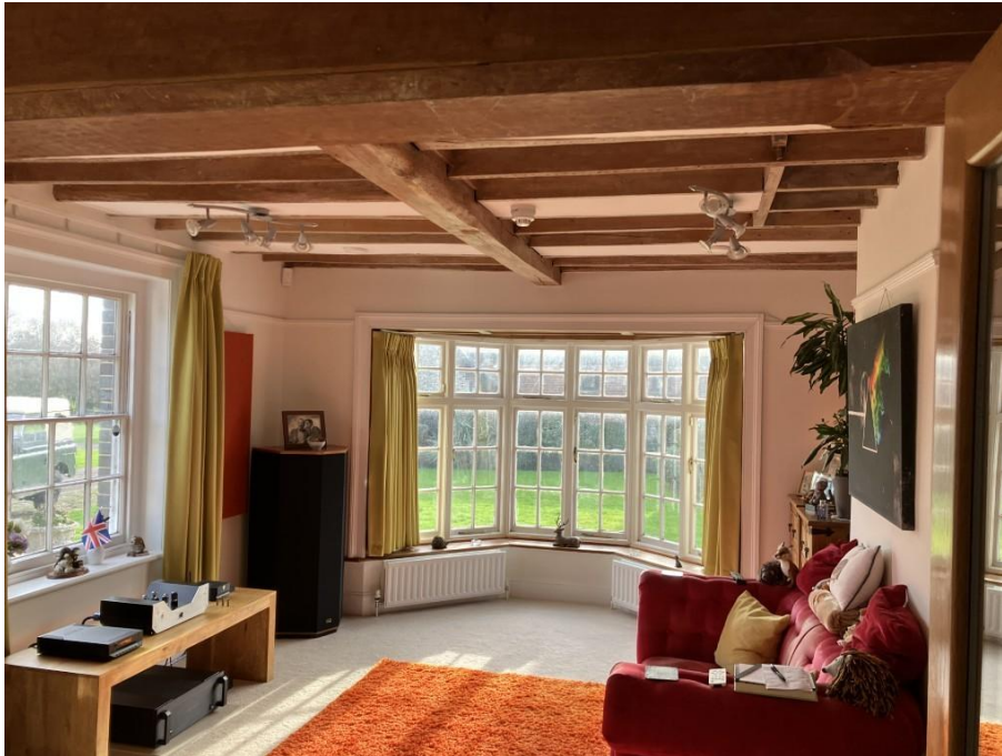
Photograph 9 – Exposed ceiling joists in current family room.
