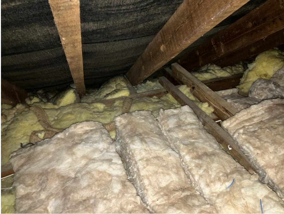
Photograph 19 – Ties over the joists appear to be lateral restraint to the hipped roof to mitigate roof spread.
