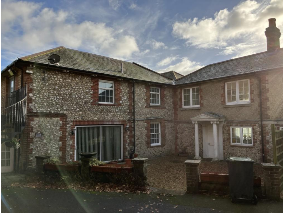
Photograph 3 – Rear/west elevation of extension and north flank wall of rear addition.
