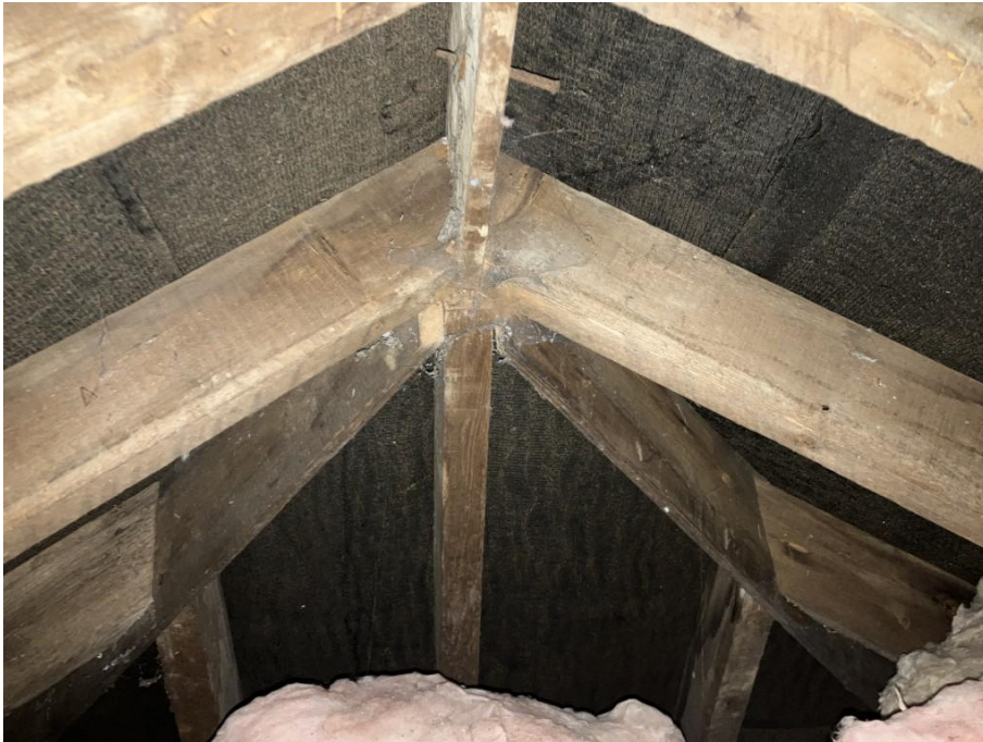
Photograph 20 – Hipped end of east end of rear addition.
