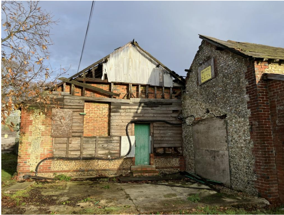
Photograph 27 – South elevation of barn with brickwork infill inside timber frame.
