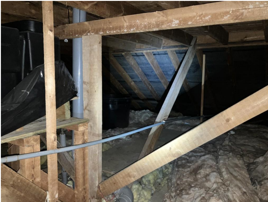
Photograph 18 – Struts support the flat roof over the extension.
