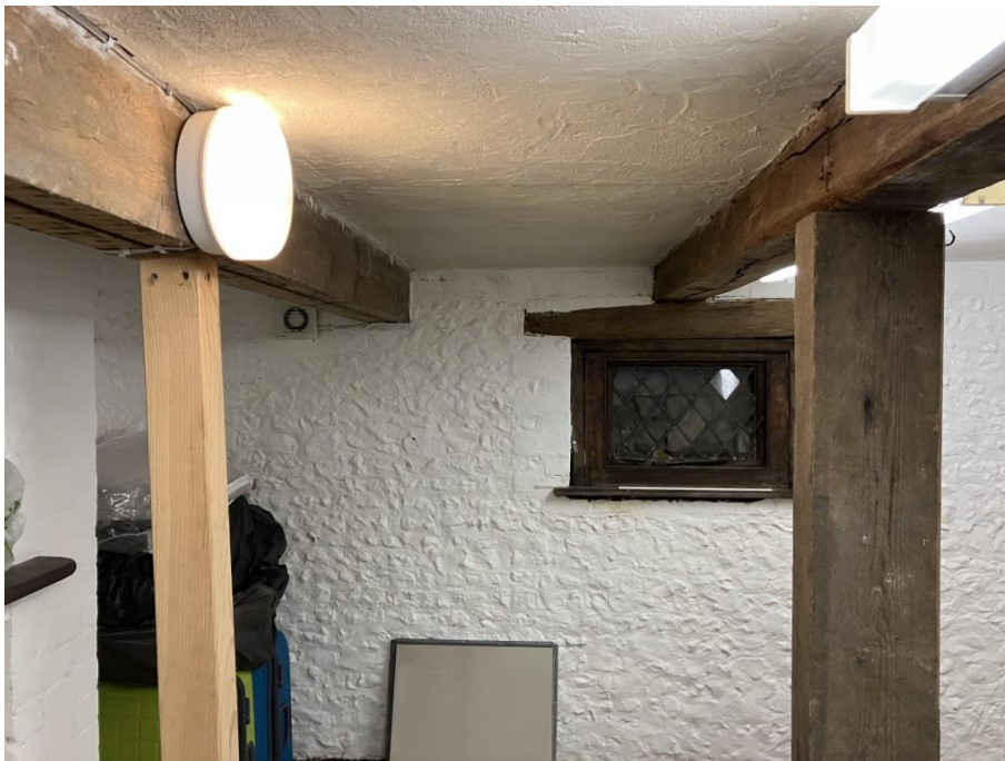
Photograph 6 – Cellar room. Left hand timbers appear to be later additions.
