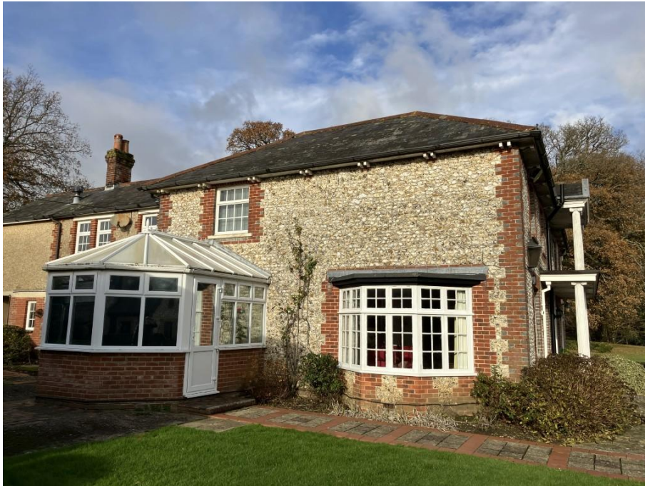
Photograph 5 – South flank wall of original house.
