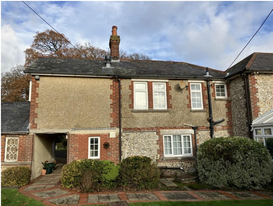
Photograph 4 – South flank wall of rear addition.
