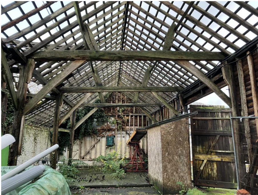
Photograph 24 – General view of barn structure looking to north.
