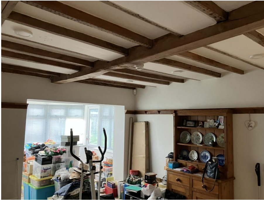
Photograph 11 – Ceiling joists exposed in ground floor south room.
