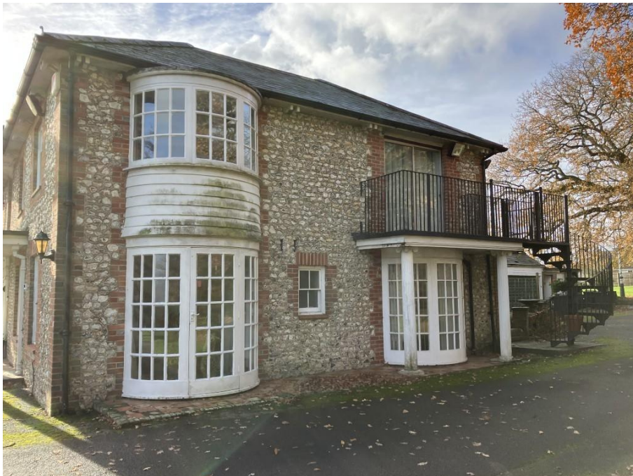
Photograph 2 – Flank/north elevation of farmhouse extension.
