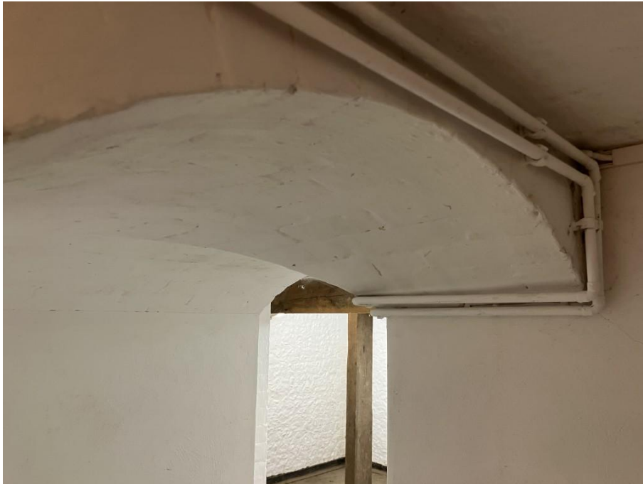
Photograph 7 – Brick arch below load bearing wall providing entrance passage to cellar.
