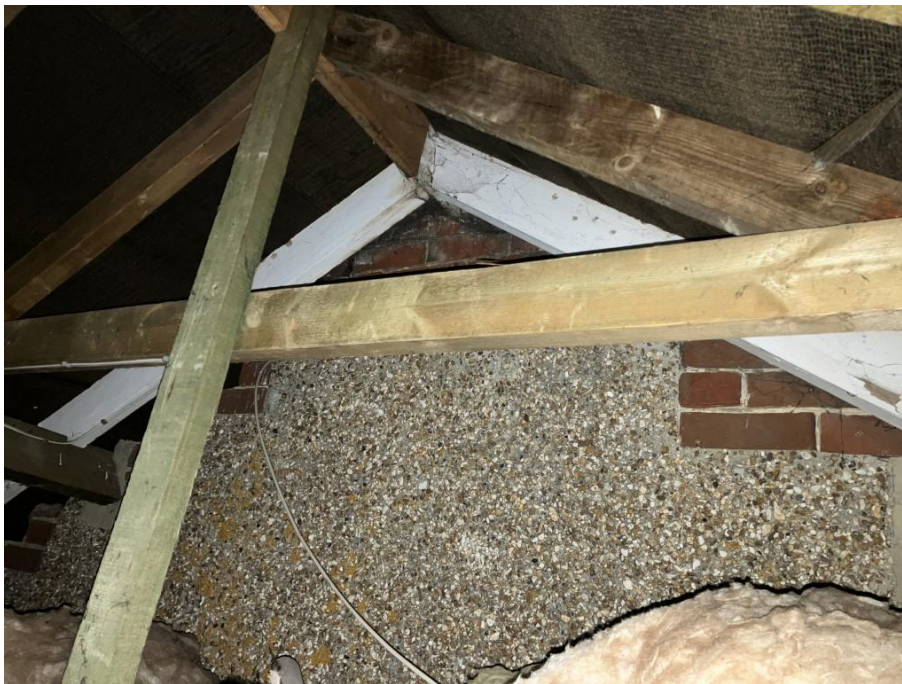
Photograph 22 – Former external pebble dash wall of rear addition in western roof void.
