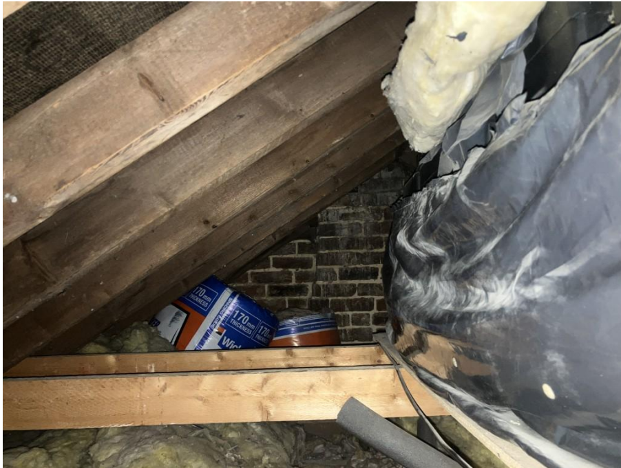
Photograph 21 – Chimney stack within east roof void of rear addition.
