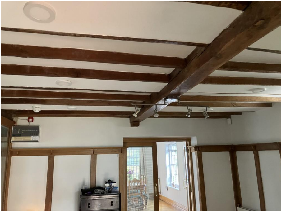
Photograph 8 – Exposed ceiling joists in current ground floor entrance hall (former front room).
