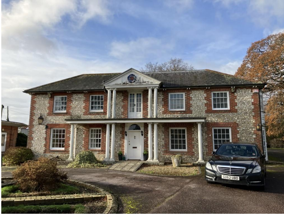
Photograph 1 – Front/east elevation of farmhouse. Left hand three bays are the original façade and the two right hand bays are the extension.
