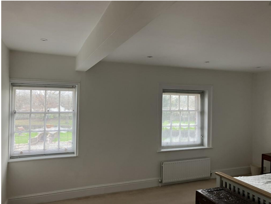
Photograph 15 – Former load bearing wall removed in first floor bedroom and replaced with a downstand beam.
