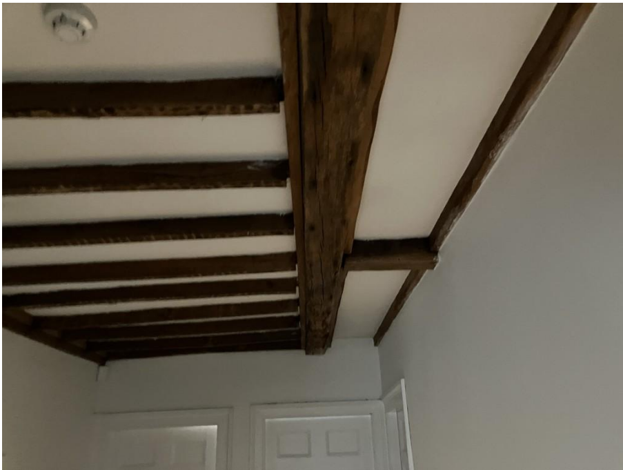
Photograph 14 – Timber beam to valley in original roof layout exposed at top of stair over first floor landing.
