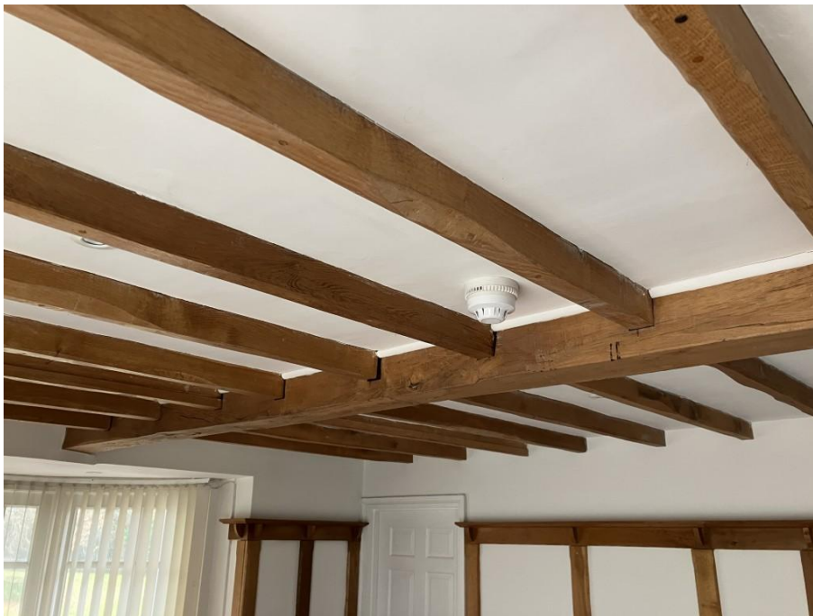
Photograph 12 – Exposed joists over ground floor rear room in extension thought to be cosmetic.
