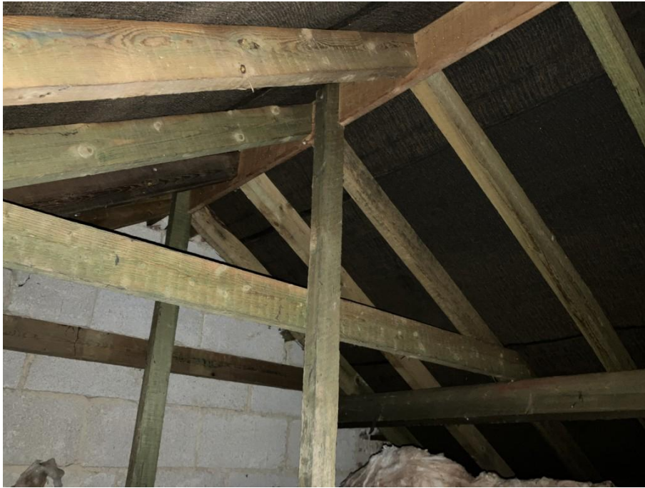
Photograph 23 – Later construction to west gable of western roof void of rear addition.
