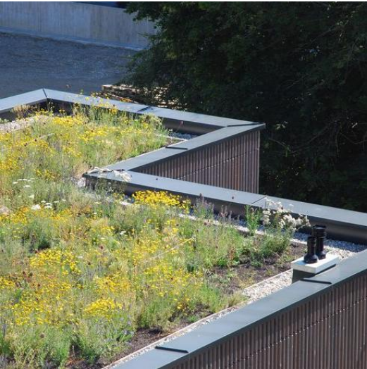
'Green' Flat Parapet Roof
