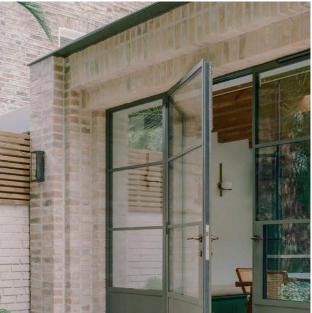
Recessed Brick Overhang Detail
