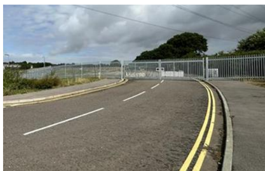
Photograph 7: Footways leading up to gated access
