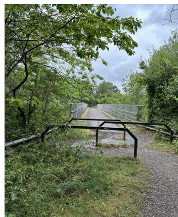
Photographs 33-34: Park Lane existing conditions heading onto bridge across A3(M) (Heading West)
