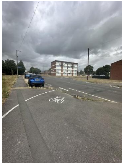
Photograph 43: Road markings on Woolston Road for cyclists to rejoin the carriageway
