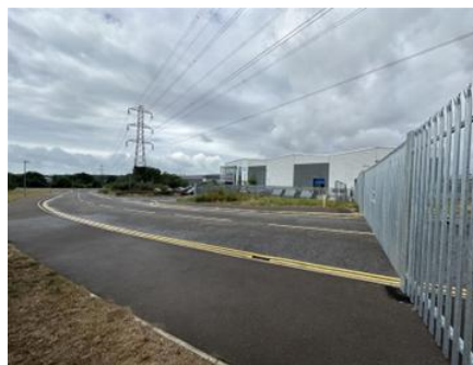
Photograph 8: Gated access to proposed Unit 400 location
