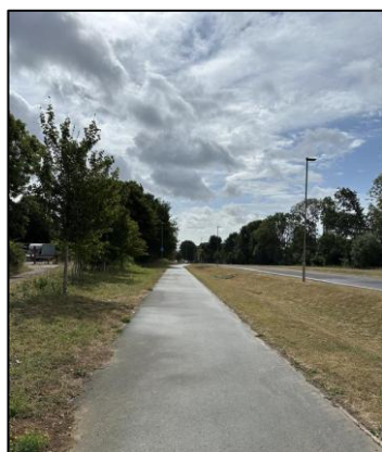
Photograph 17: Footway connection on the northern side of the carriageway towards Woolston Road (Heading East from Dunsbury Park)
