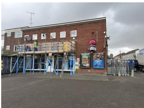
Photograph 48: One Stop on Middle Park Way
