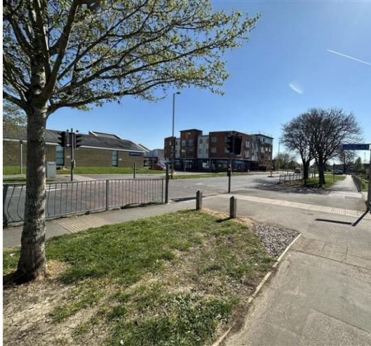
Photograph 56: Toucan Crossing on Dunsbury Way (looking south-east)
