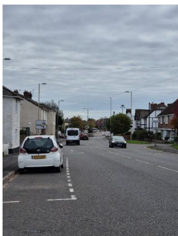
Photograph 82: Existing conditions on Bedhampton Road (B2149)
