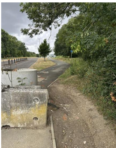
Photograph 19: Footway on Fitzwygram Way heading towards Woolston Road (Facing west towards Dunsbury Park)
