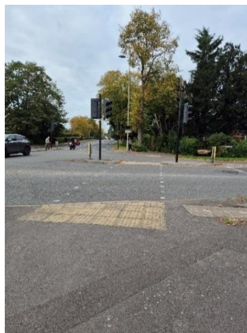
Photograph 81: Signalised crossing across Hulbert Road (B2150)
