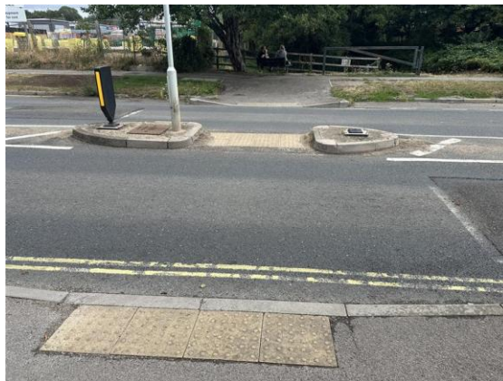
Photograph 54: Crossing point on Dunsbury Way
