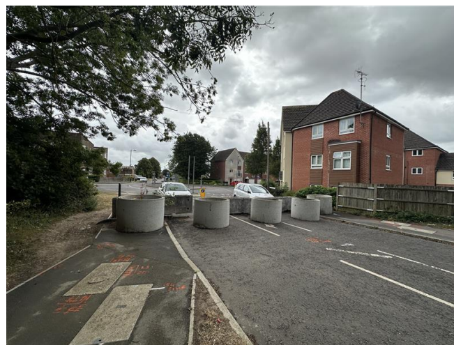
Photograph 20: Bollards to the south of Dunsbury Park near the roundabout (Calshot Road/Woolston Road/Freeley Road/Fitzwygram Way) & where Fitzwygram Way shared footway/cycleway terminates
