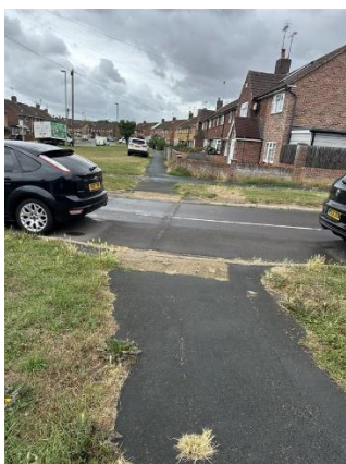
Photograph 60: Crossing point on Park House Farm Way heading towards Purbrook Way (western side of the carriageway across Quarely Road)
