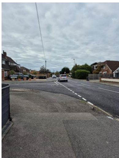
Photograph 77: Existing Conditions near Hooks Lane
