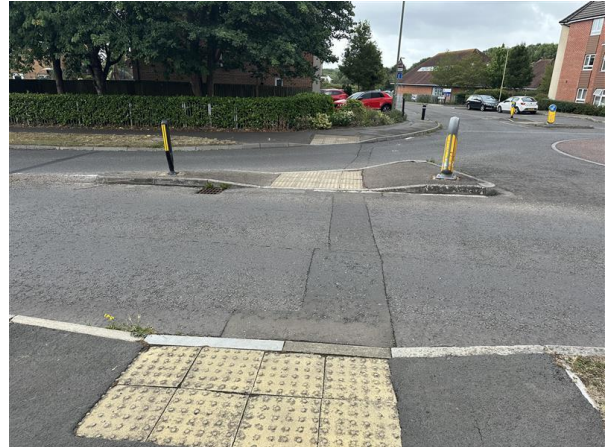
Photograph 22: Crossing Point on the roundabout (Calshot Road/Woolston Road/Freeley Road/Fitzwygram Way) Woolston Road
