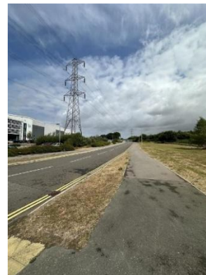
Photograph 12: Existing Conditions on Fitzwygram Way (West of the proposed site on the southern side of the carriageway)
