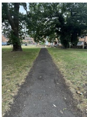
Photograph 59: Footway between Middle Park Way and Park House Farm Way.
