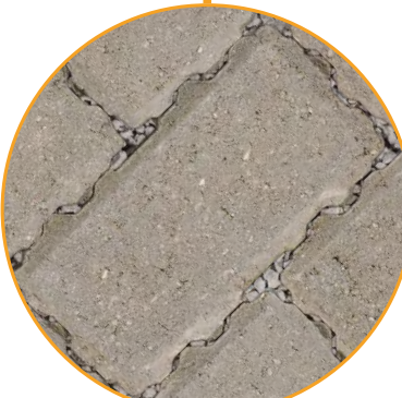
Paved Footpath Marshalls Block Paving
