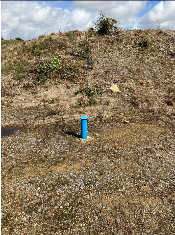
Figure 8: Monitoring well at base of soil bund
