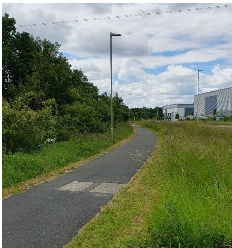
Photograph 4: Footway on southern side of Fitzwygram Way.
