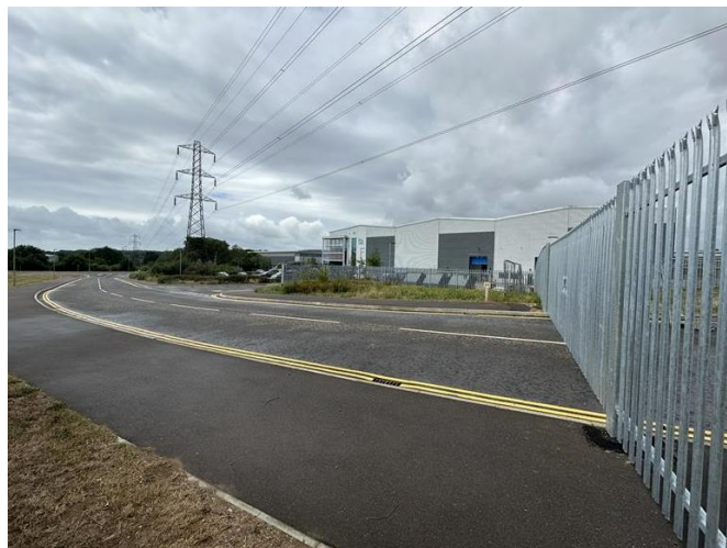
Photograph 1: Gated access to proposed Unit 400 location
