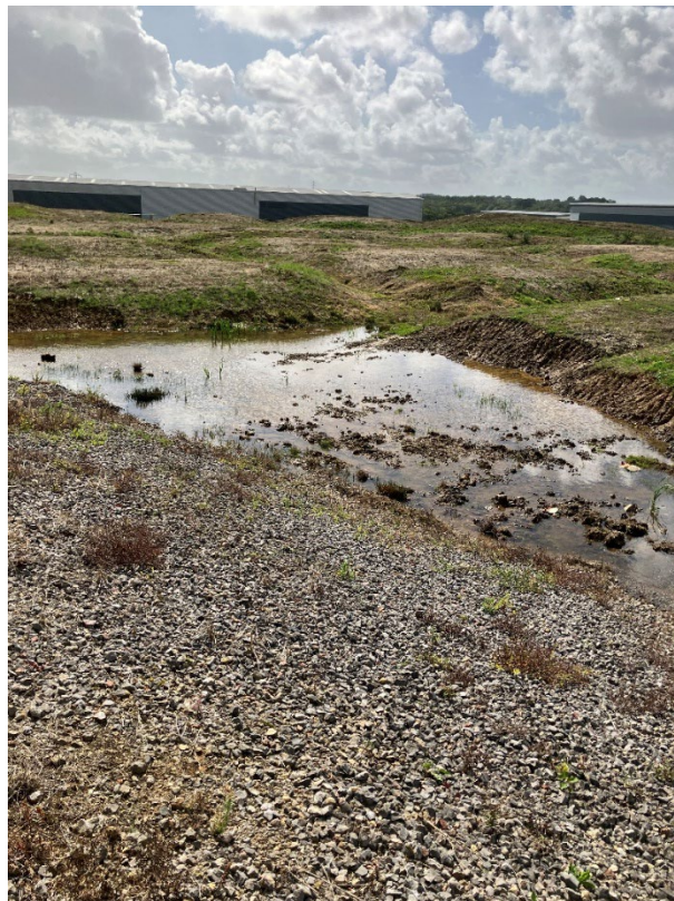
Figure 14: Ponding water between soil stockpiles
