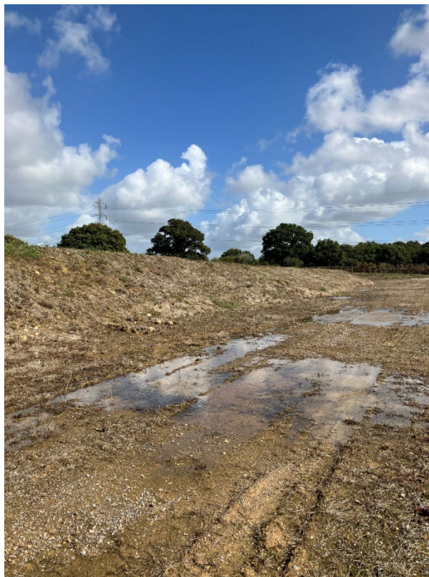
Figure 7: Looking NE, note 3m high soil bund
