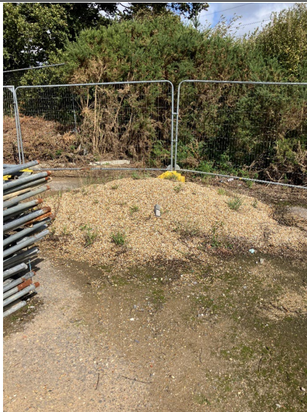
Figure 16: Heras fencing and pea gravel stockpile along eastern boundary
