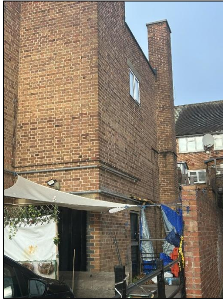
Photograph 18: Proposed pedestrian entrance to the site
