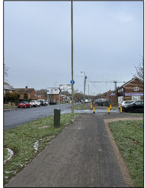
Photograph 8: Shared footway/cycleway on Dunsbury Way
