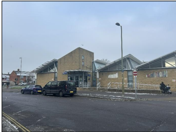
Photograph 7: Leigh Park Library and shared footway/cycleway on northern side of Park Parade
