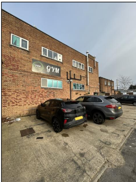
Photograph 1: Site rear forecourt
