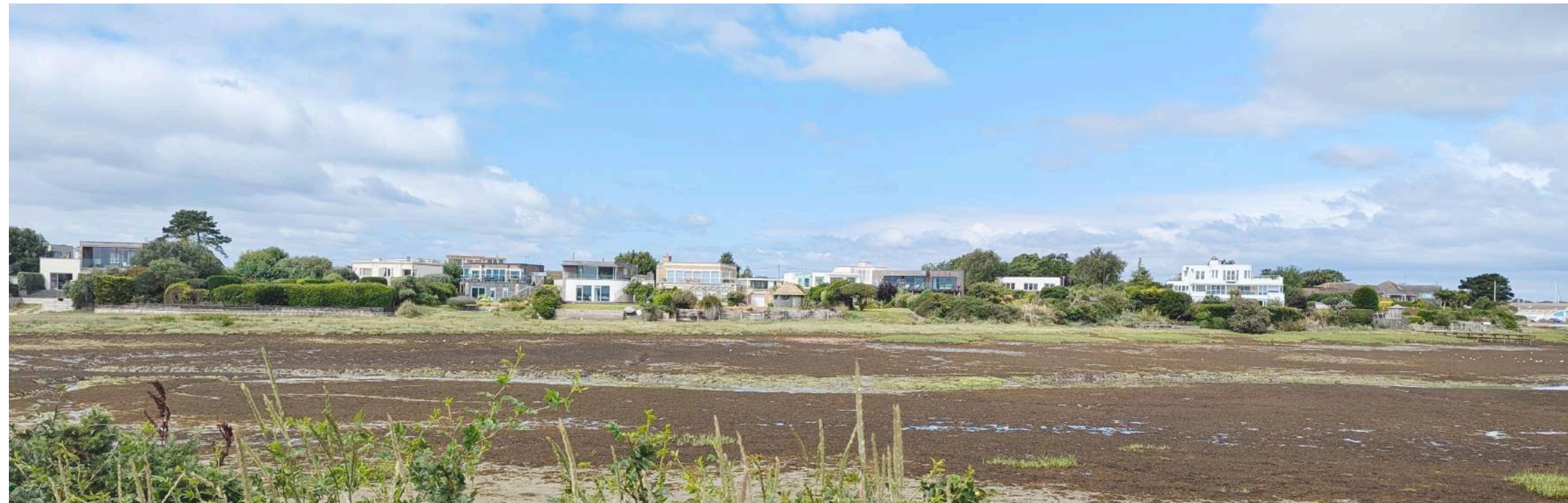
Rear view of 2 - 26 Wittering Road
