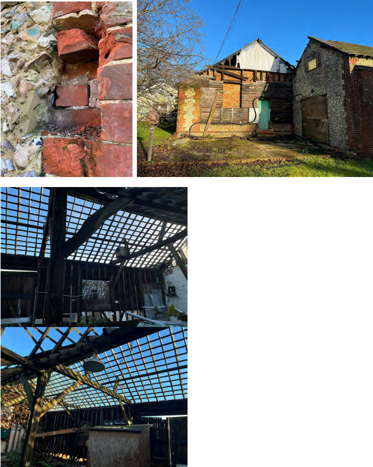
Plate 2: 19 th Century Shed (Building 05) existing condition. Details (19 December 2025)
