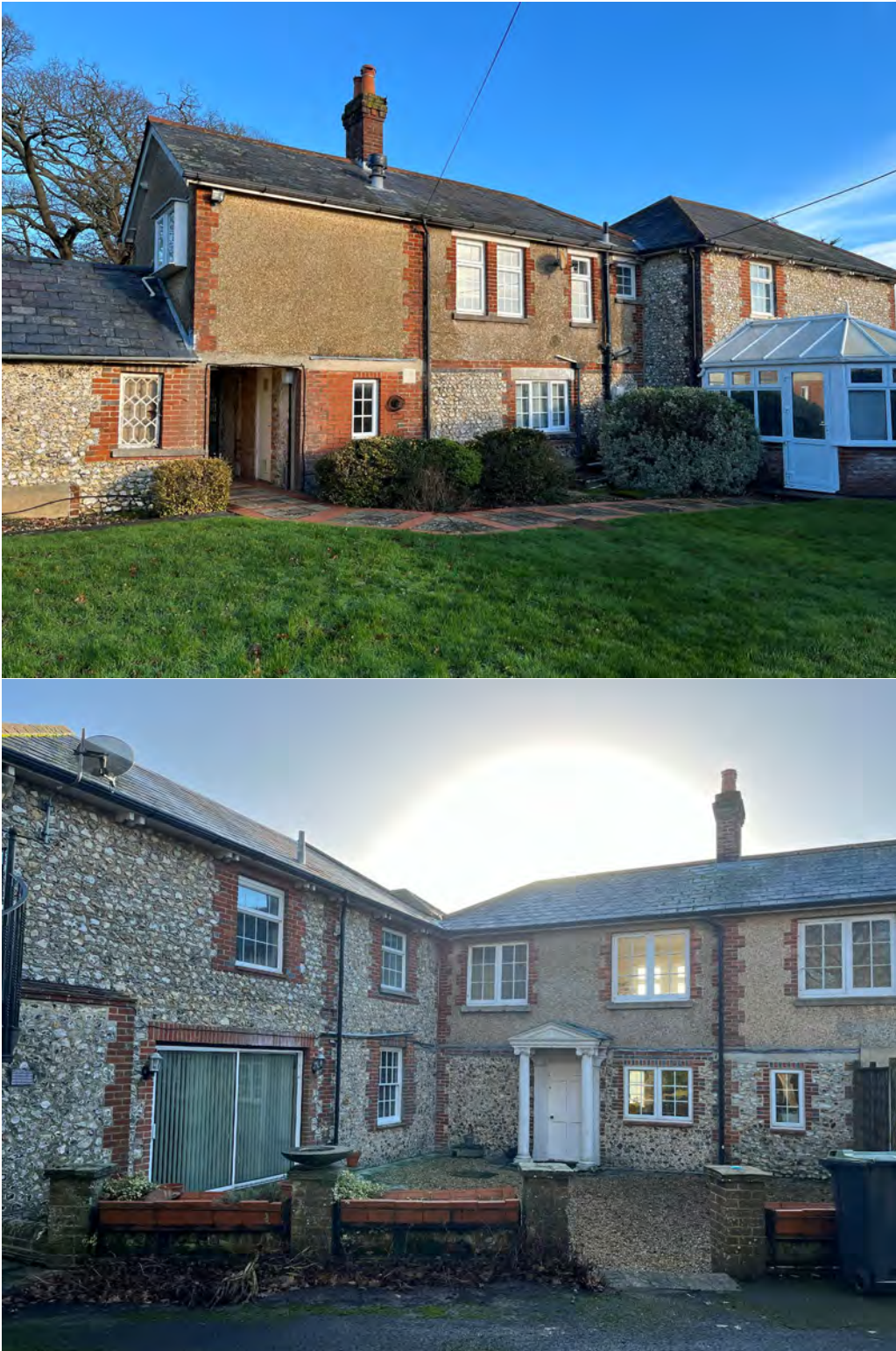
Plate 4: Farmhouse existing condition (19 December 2025)
