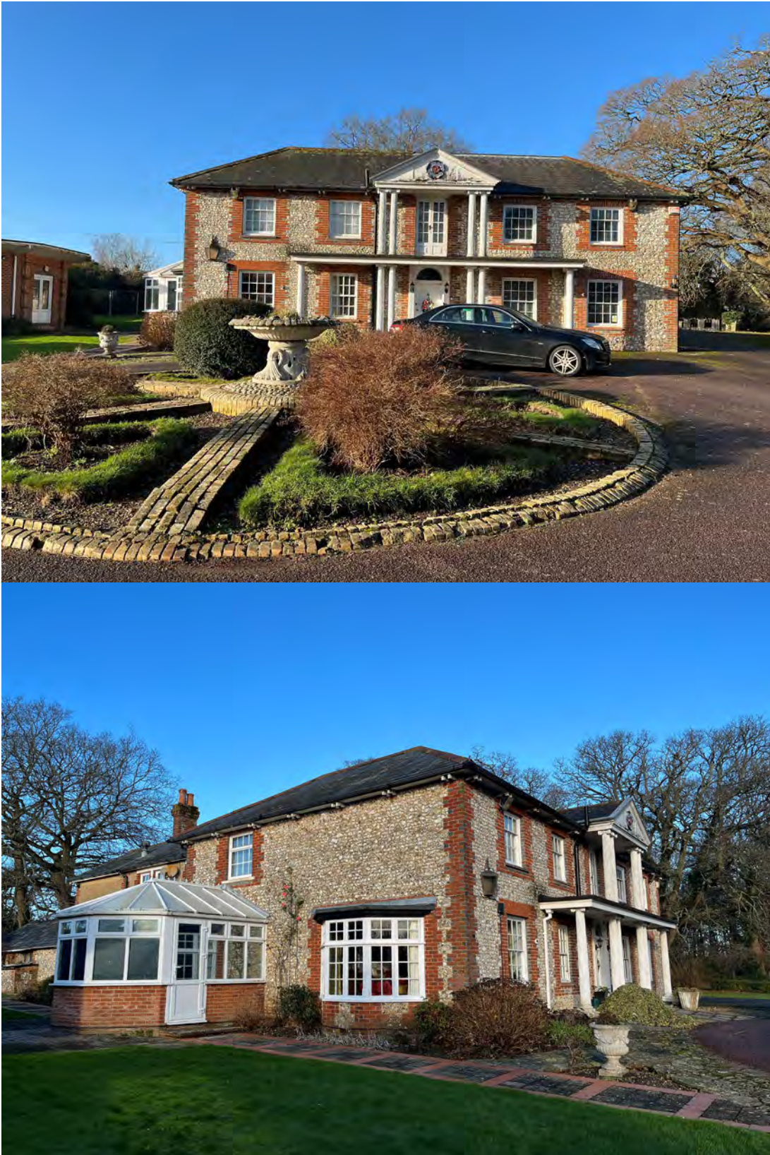
Plate 3. Padnell Grange Farmhouse (Building 01) existing condition (19 December 2025)
