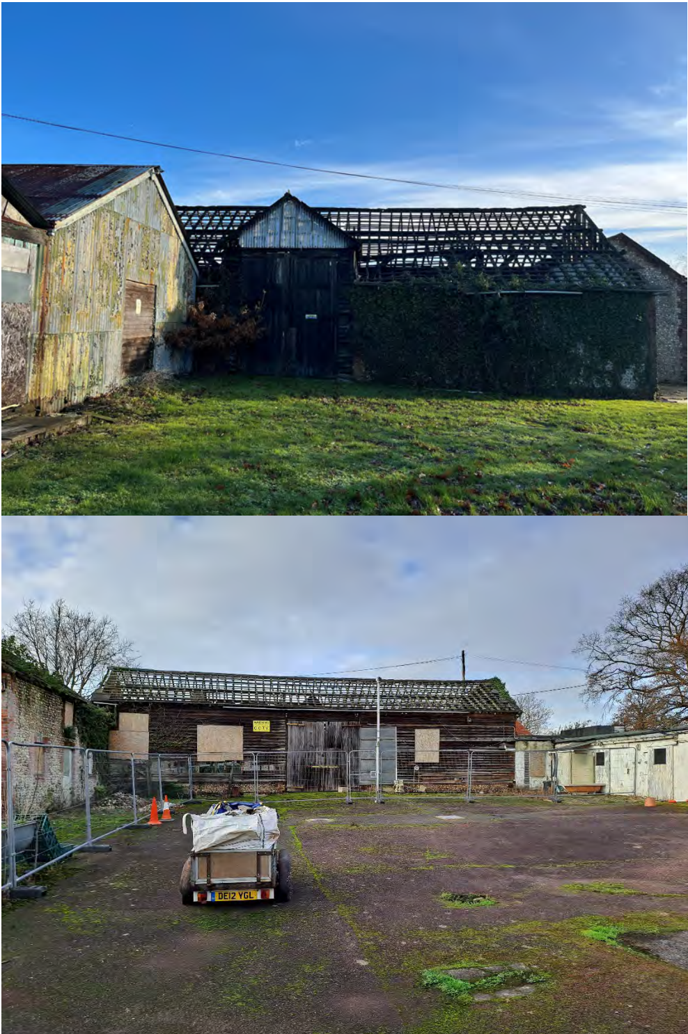
Plate 1: 19 th Century Shed existing condition (19 December 2025)
