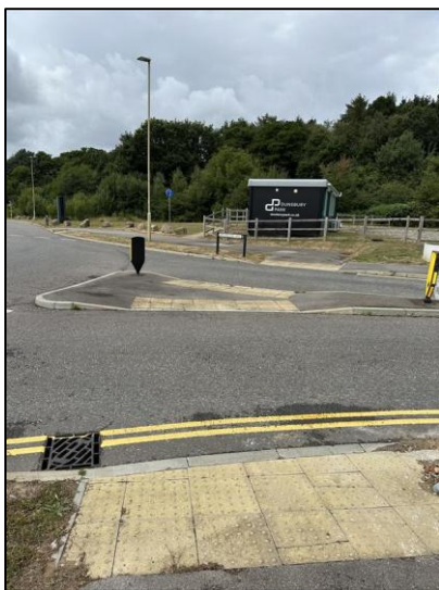
Photograph 6: Pedestrian Crossing Point within Dunsbury Park across the roundabout (north of proposed site)
