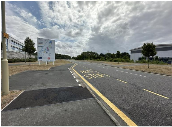
Photograph 10: Bus stop on Fitzwygram Way (Eastbound)
