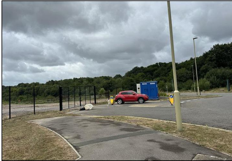
Photograph 1: Access to Unit 100 from the roundabout (looking west)
