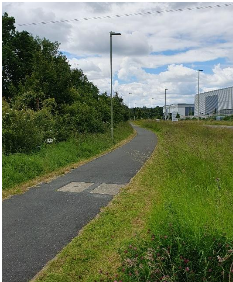
Photograph 4: Footway on southern side of Fitzwygram Way.
