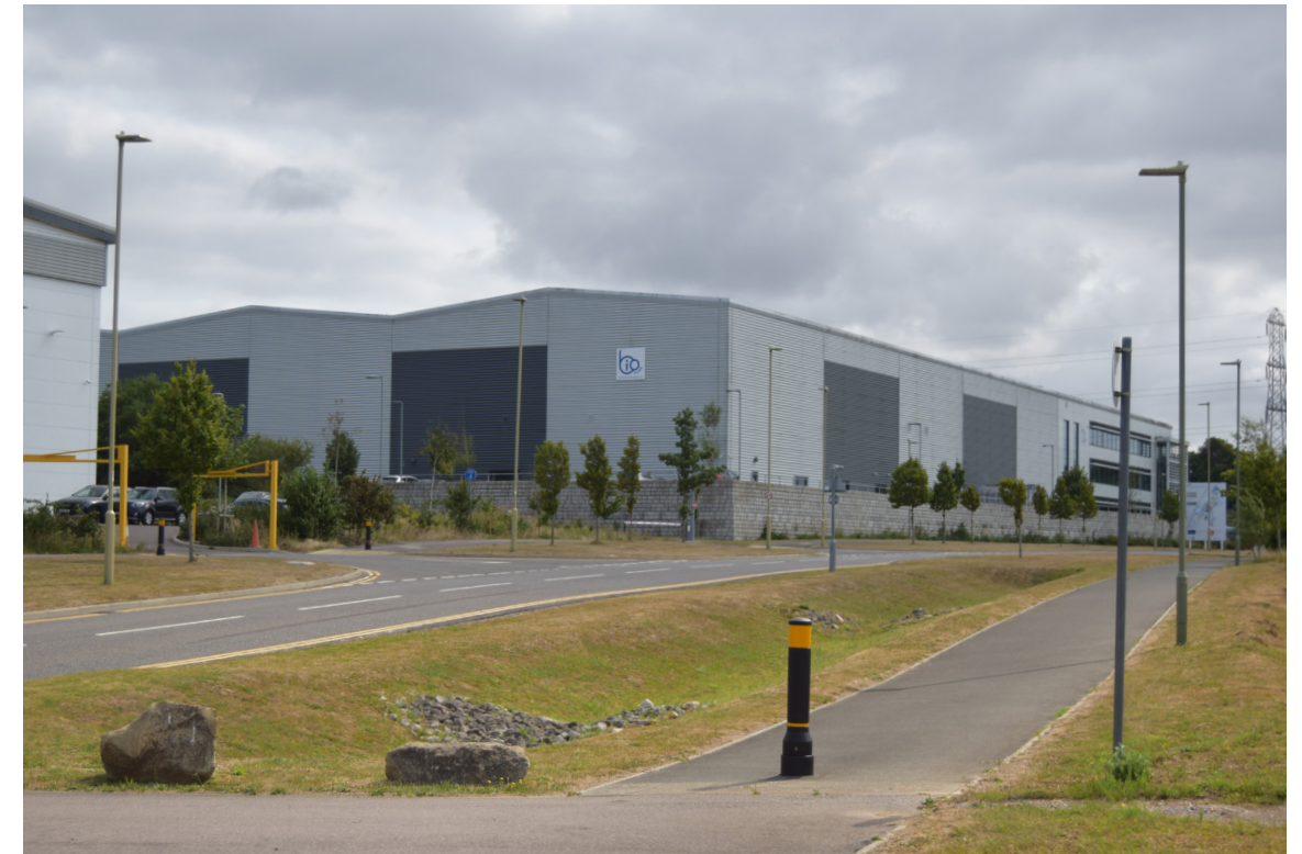
Looking east along Fitzwygram Way. Plots 400 and 600 lie beyond the building.
