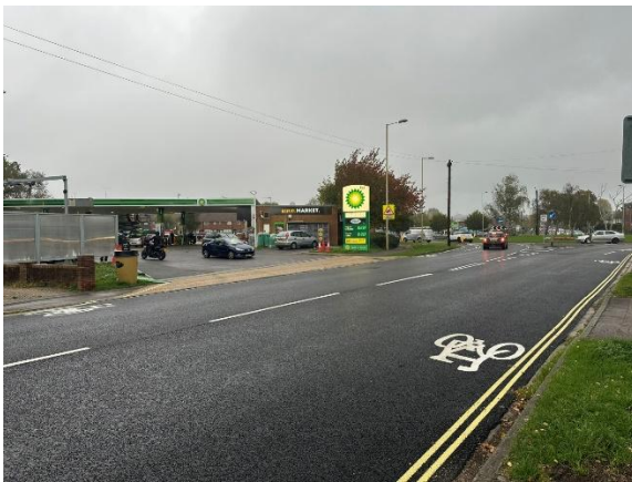
Photograph 72: Cycle lanes terminate on Park Lane – looking north
