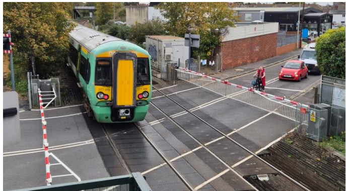
Photograph 85: A cyclist utilising the carriageway to cross the train track.
