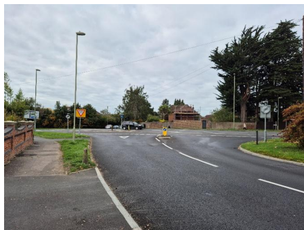
Photograph 77: Existing Condition heading towards Hulbert Road (B2150)
