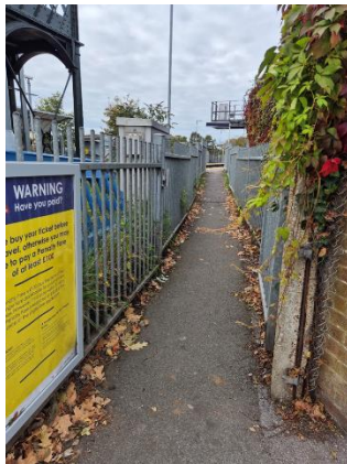
Photograph 84: Access to Platform 1
