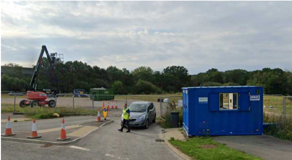
02 North view into Plot 100 from entrance
