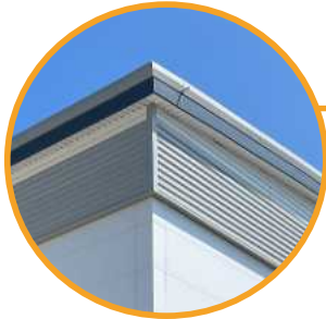
Built up horizontally laid trapezoidal profile metal wall cladding system Finish: Tata Colorcoat HPS200 Ultra Colour: Goosewing Grey (RAL 7038)
