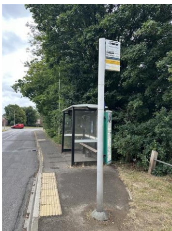
Photograph 25: Footway and bus stop condition on Calshot Road (Southern edge of carriageway)
