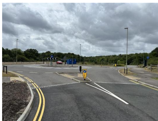
Photograph 8: Roundabout on Fitzwygram Way (Facing the access of Unit 100 to the south)
