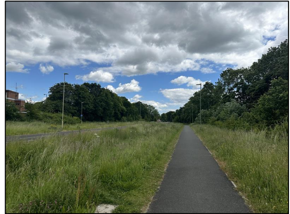
Photograph 17: Footway connection on the southern side of the carriageway towards Woolston Road (Heading East from Dunsbury Park)
