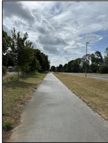
Photograph 16: Footway connection on the northern side of the carriageway towards Woolston Road (Heading East from Dunsbury Park)
