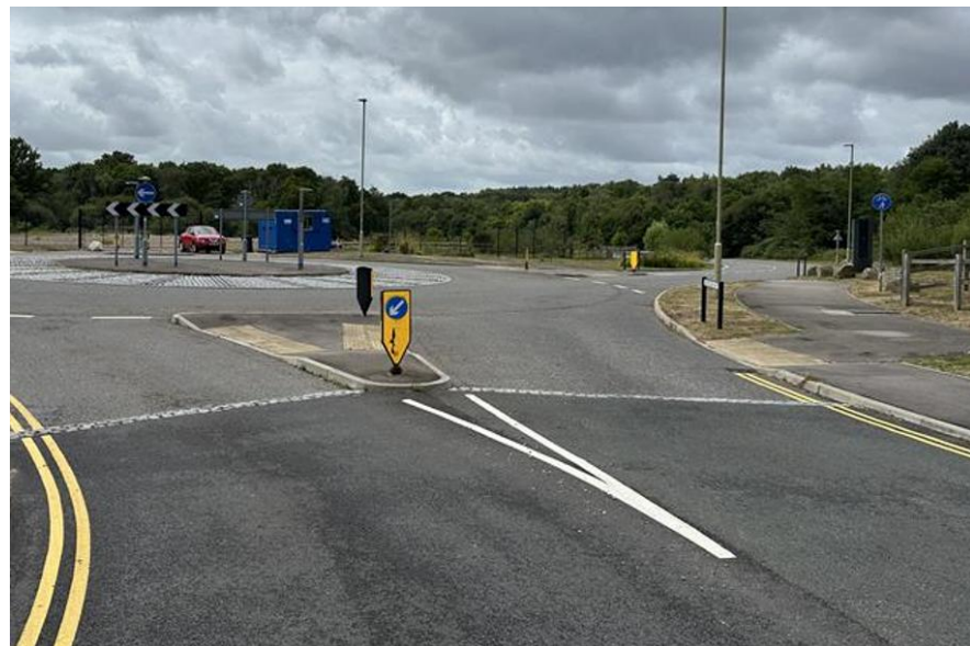
Photograph 11: Conditions of the roundabout showing where footway/cycleway terminates to the west
