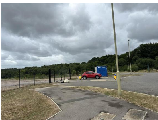
Photograph 7: Existing access for Unit 100 location
