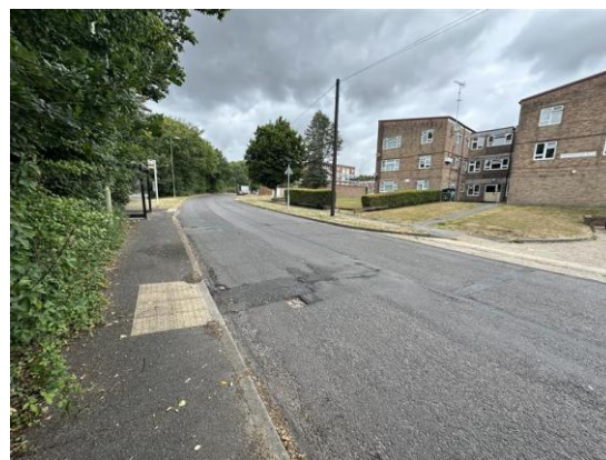
Photograph 26: Footway leading to the bus stop on Calshot Road & crossing point across carriageway (Southern edge of carriageway)
