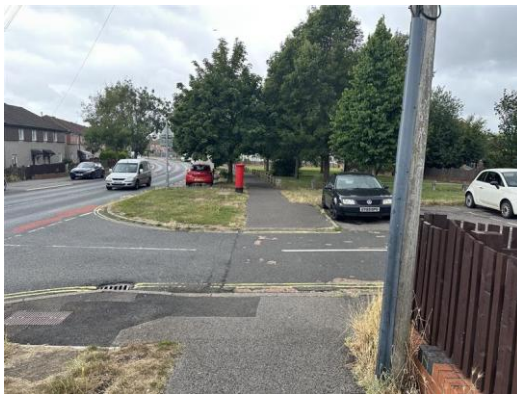
Photograph 46: Dropped kerbs across Locksheath Close junction on Middle Park Way
