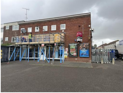
Photograph 47: One Stop on Middle Park Way
