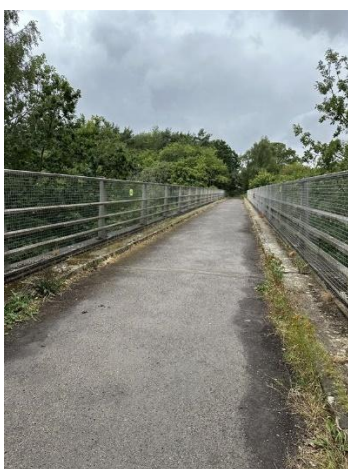
Photograph 34: Park Lane existing conditions heading over the bridge
