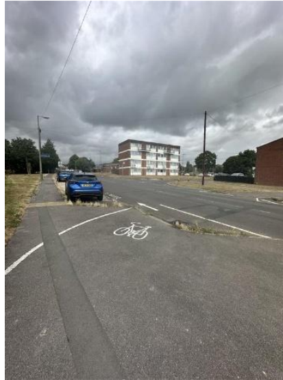
Photograph 42: Road markings on Woolston Road for cyclists to rejoin the carriageway
