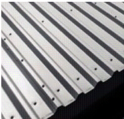
1 METAL BUILT UP ROOF CLADDING IN GOOSEWING GREY (RAL 7038).
