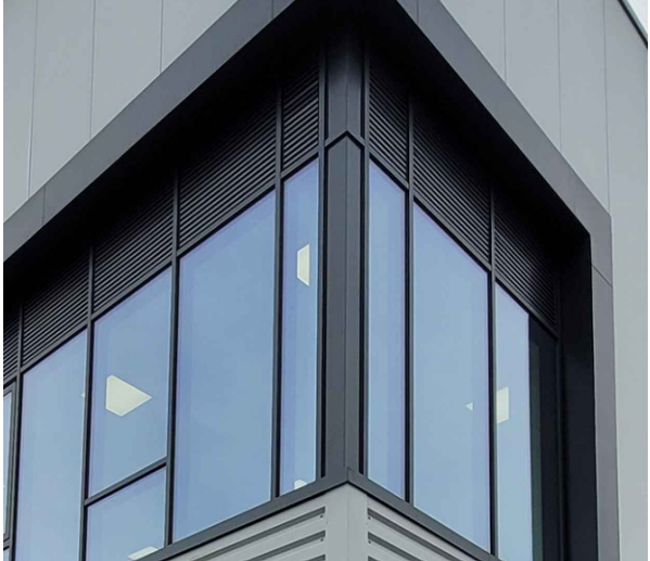
6 7 ALUMINIUM FRAMED GLAZING IN ANTHRACITE GREY (RAL 7016).
