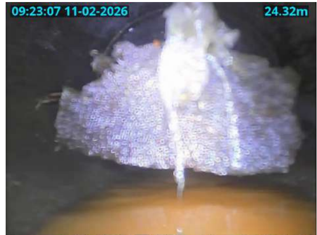
MH38X_U_11022026_0923_078.jpg, 00:02:27, 24.32 m Survey abandoned, Overlap complete
