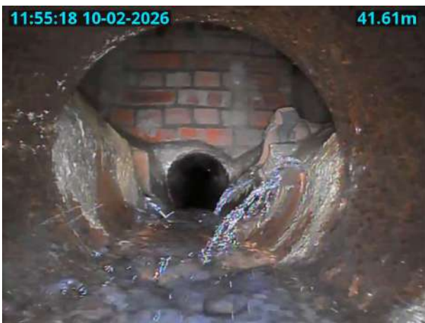
MH10X_U_10022026_1155_050.jpg, 00:05:22, 41.61 m General remark, Heavy infiltraton from MH
