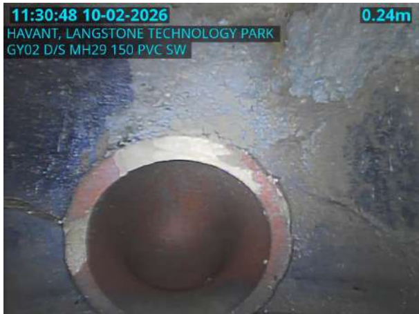
GY2X_D_10022026_1130_046.jpg, 00:00:07, 0.24 m Finish node, manhole, reference: MH29
