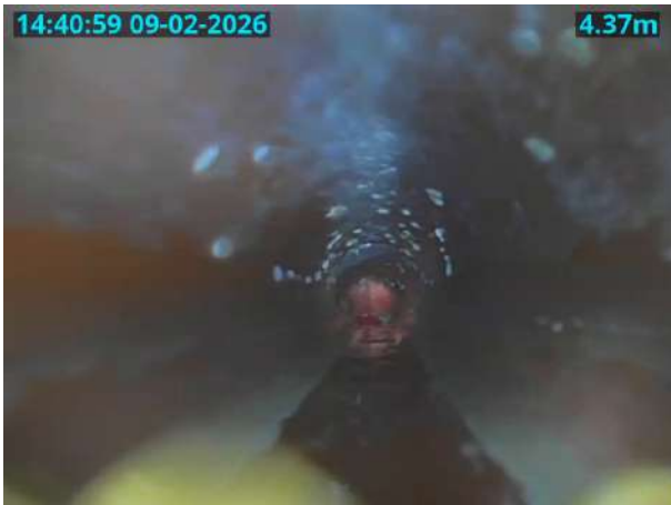
MH15X_D_09022026_1441_097.jpg, 00:00:27, 4.37 m General photograph taken at this point
