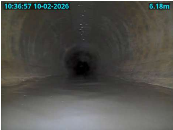
MH23X_D_10022026_1042_041.jpg, 00:00:59, 6.18 m General photograph taken at this point
