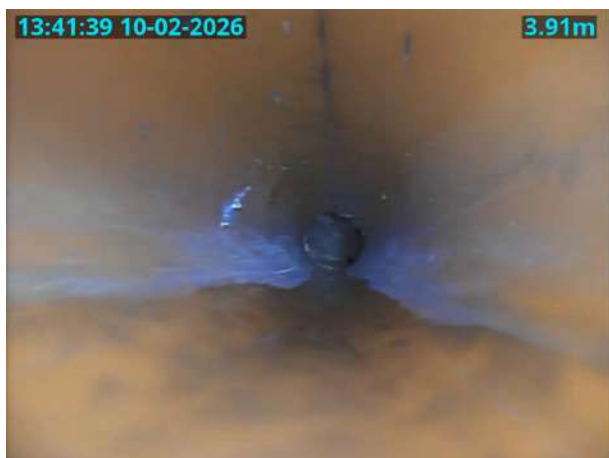
MH32AX_U_10022026_1341_054.jpg, 00:00:25, 3.91 m General photograph taken at this point
