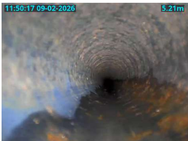
MH8X_D_09022026_1151_012.jpg, 00:00:40, 5.21 m General photograph taken at this point
