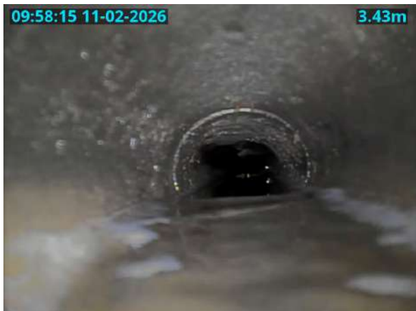
MH41X_D_11022026_0958_112.jpg, 00:00:20, 3.43 m General photograph taken at this point
