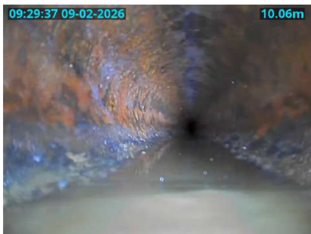
MH1X_D_09022026_0934_001.jpg, 00:01:21, 10.06 m General photograph taken at this point
