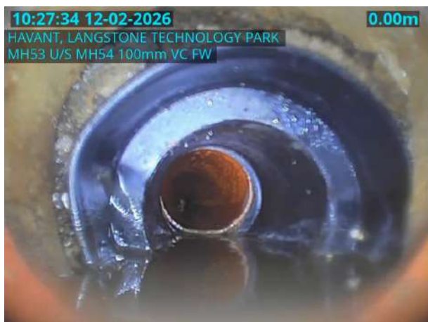
MH54X_798307c4-09e6-4b34-a5a9-306f880723f1_20260223_125610_257.jpg, 00:00:03, 0.00 m Water level, 20% of the vertical dimension
