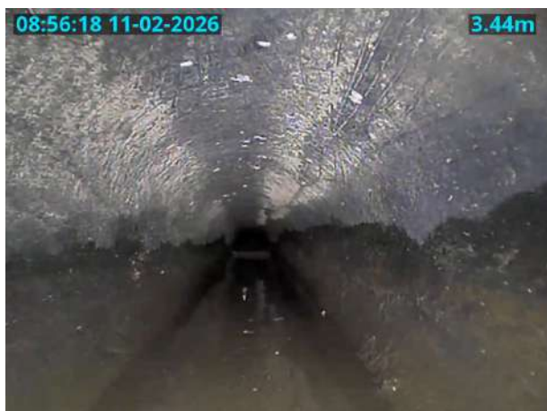
MH38X_D_11022026_0856_072.jpg, 00:00:43, 3.44 m General photograph taken at this point
