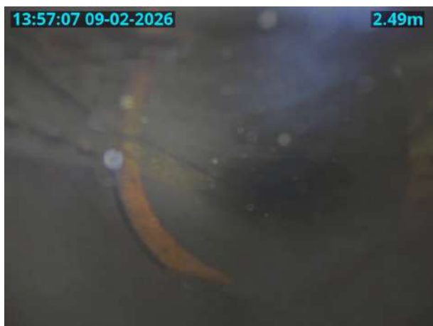
10BX_U_09022026_1357_019.jpg, 00:00:18, 2.49 m Joint displaced, medium, Visible through water
