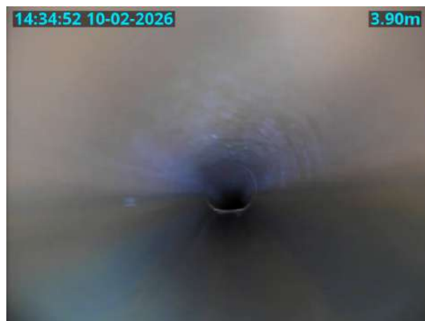
36AX_U_10022026_1435_064.jpg, 00:00:20, 3.90 m General photograph taken at this point
