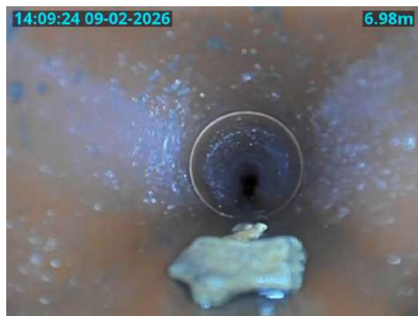
12AX_U_09022026_1411_023.jpg, 00:00:47, 6.98 m General photograph taken at this point
