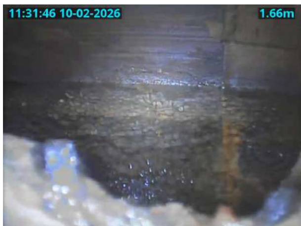
MH29X_D_10022026_1131_047.jpg, 00:00:14, 1.66 m Finish node, major connection without manhole, reference: Main
