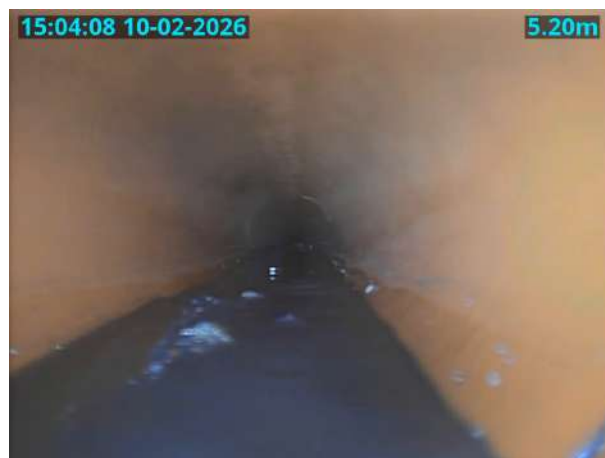
MH37X_D_10022026_1505_070.jpg, 00:00:37, 5.20 m General photograph taken at this point
