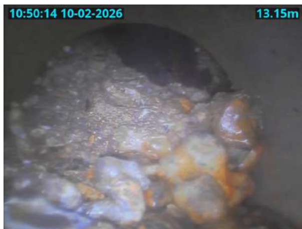
MH26X_U_10022026_1050_043.jpg, 00:01:20, 13.15 m Finish node, other special chamber, reference: MH26, Pipe runs to ground
