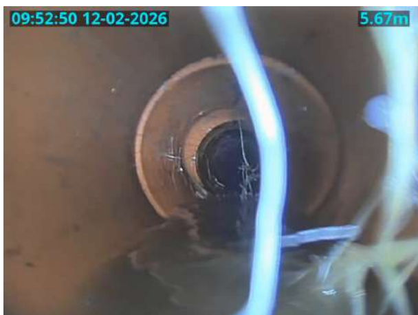
MH50X_501639b4-1eef-4419-a24c-3575b4543346_20260223_123148_407.jpg, 00:00:45, 5.67 m Roots, mass, 10% cross-sectional area loss
