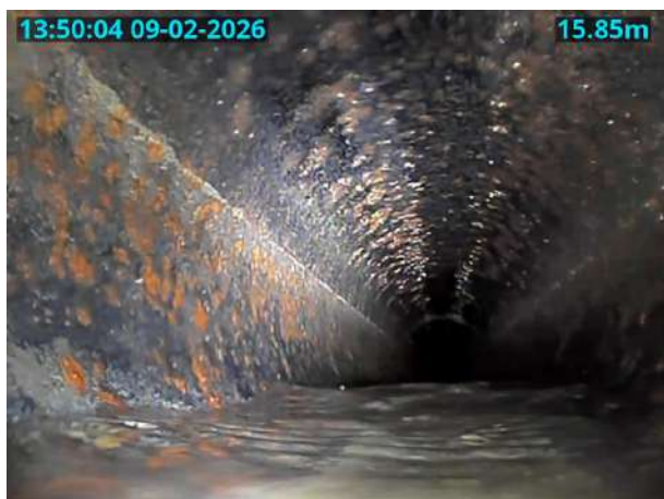
10AX_U_09022026_1352_017.jpg, 00:01:59, 15.85 m General photograph taken at this point
