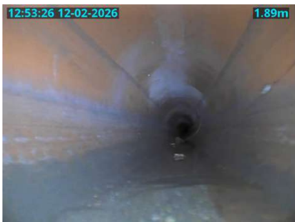
MH72X_c1071194-29da-4955-a7d5-f5be990bfeba_20260223_141356_370.jpg, 00:00:19, 1.89 m Settled deposits, fine, 5% cross-sectional area loss, start
