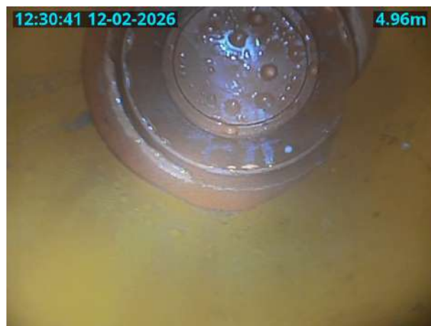
67AX_694923d4-9b3e-47ff-87b4-f1e0f30c1e9e_20260223_140410_886.jpg, 00:00:36, 4.96 m Finish node, other special chamber, reference: 67A, CAPPED OFF
