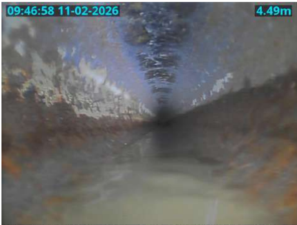
MH33CX_D_11022026_0947_082.jpg, 00:00:32, 4.49 m General photograph taken at this point
