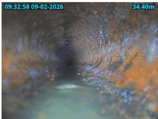
MH1X_D_09022026_0934_003.jpg, 00:04:42, 34.40 m General photograph taken at this point
