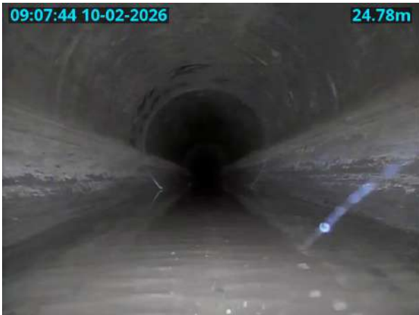
MH21X_D_10022026_0908_039.jpg, 00:03:11, 24.78 m General photograph taken at this point
