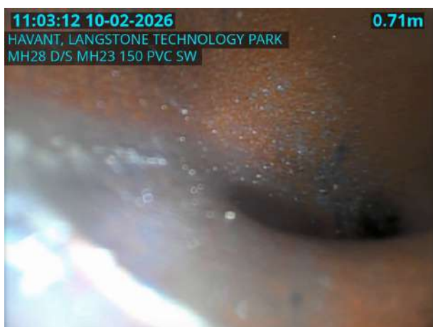
MH28X_D_10022026_1103_044.jpg, 00:00:07, 0.71 m General photograph taken at this point
