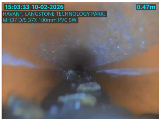
MH37X_D_10022026_1505_069.jpg, 00:00:02, 0.47 m General photograph taken at this point
