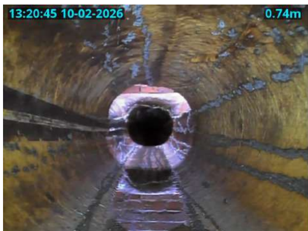
MH32X_D_10022026_1320_052.jpg, 00:00:11, 0.74 m General photograph taken at this point
