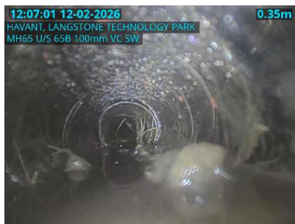
65BX_6caa402f-0d17-43a1-84e7-f25ef14caea4_20260223_134908_595.jpg, 00:00:06, 0.35 m Roots, fine
