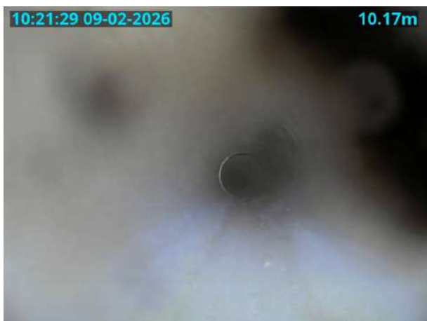
4AX_U_09022026_1025_087.jpg, 00:01:32, 10.17 m General photograph taken at this point
