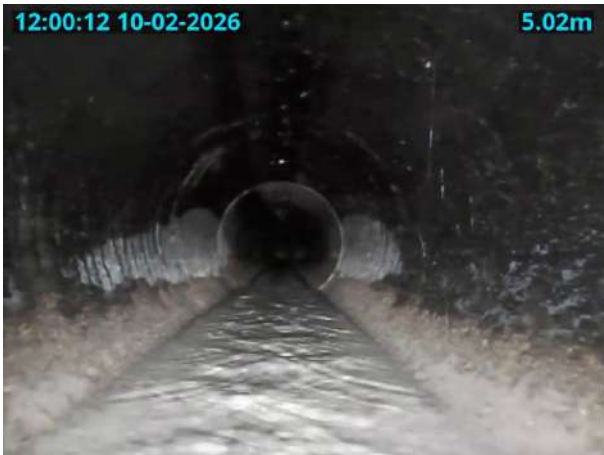
MH30X_D_10022026_1201_106.jpg, 00:00:35, 5.02 m General photograph taken at this point
