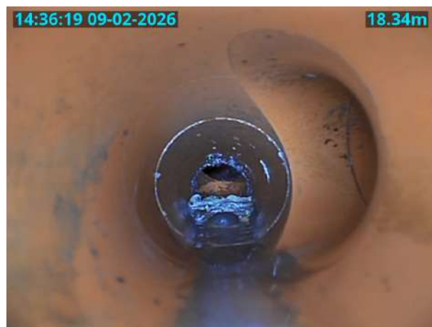
14AX_U_09022026_1436_032.jpg, 00:01:48, 18.34 m General photograph taken at this point
