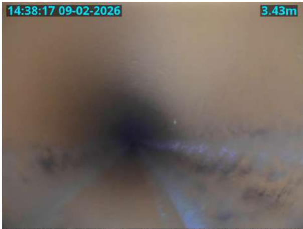
MH14X_D_09022026_1439_033.jpg, 00:00:23, 3.43 m General photograph taken at this point
