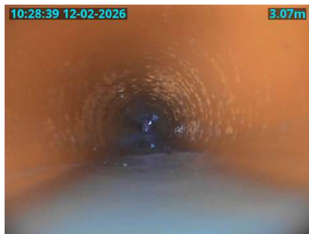
MH54X_2803b975-b308-4e8e-83bb-015ae72626ca_20260223_125645_123.jpg, 00:01:07, 3.07 m Water level, 5% of the vertical dimension
