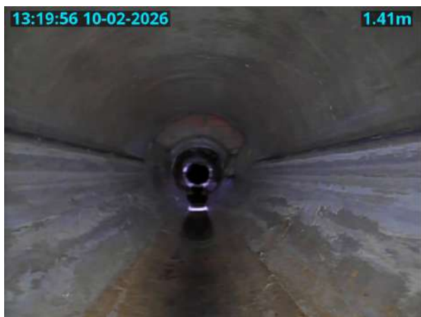
MH31X_D_10022026_1320_051.jpg, 00:00:19, 1.41 m General photograph taken at this point
