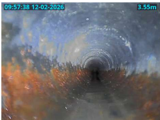
50AX_d744a6ec-30cf-4855-887a-bebf4297be33_20260223_1 23910_965.jpg, 00:00:29, 3.55 m General photograph taken at this point
