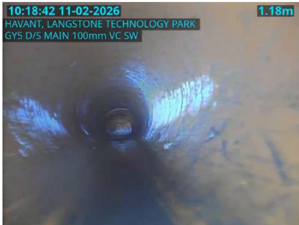
GY5X_D_11022026_1018_085.jpg, 00:00:07, 1.18 m General photograph taken at this point
