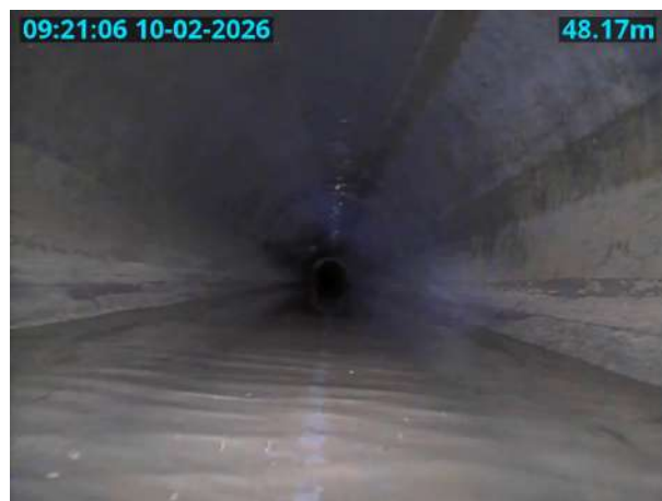
MH22X_D_10022026_0921_105.jpg, 00:05:34, 48.17 m General photograph taken at this point
