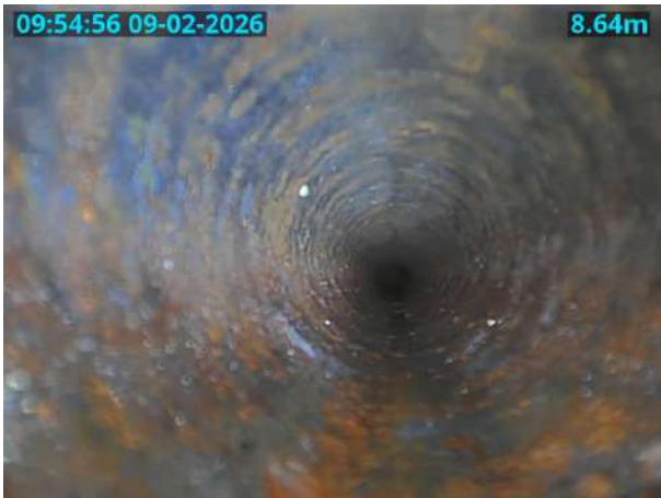
2AX_U_09022026_0955_005.jpg, 00:01:35, 8.64 m General photograph taken at this point
