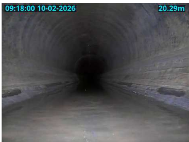
MH22X_D_10022026_0921_104.jpg, 00:02:29, 20.29 m General photograph taken at this point
