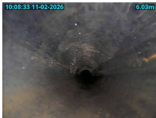
GY4X_D_11022026_1009_084.jpg, 00:00:40, 6.03 m General photograph taken at this point
