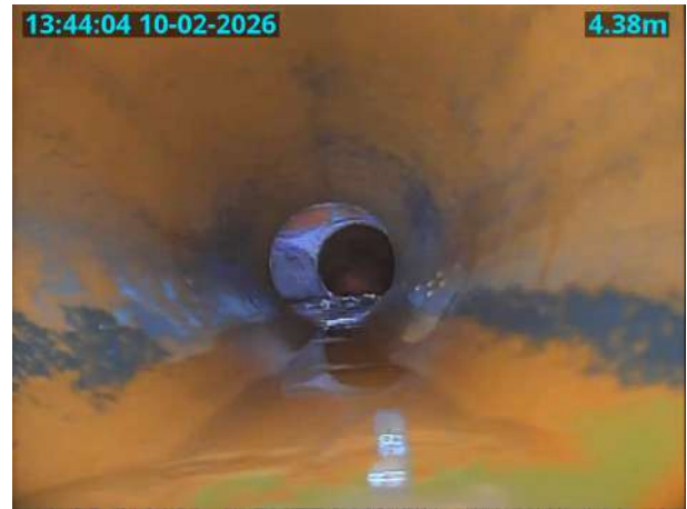
MH32AY_U_10022026_1344_056.jpg, 00:00:25, 4.38 m General photograph taken at this point
