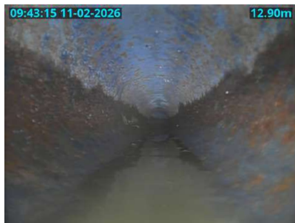
MH40X_D_11022026_0943_081.jpg, 00:01:27, 12.90 m General photograph taken at this point
