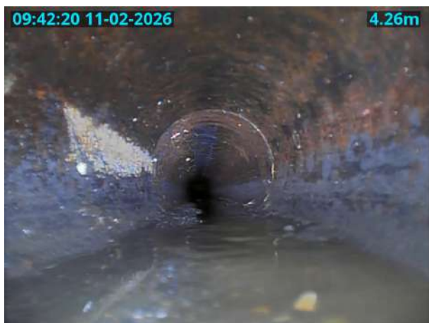
MH40X_D_11022026_0943_080.jpg, 00:00:31, 4.26 m General photograph taken at this point
