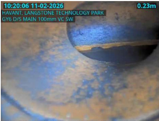
GY6X_D_11022026_1020_086.jpg, 00:00:03, 0.23 m General photograph taken at this point
