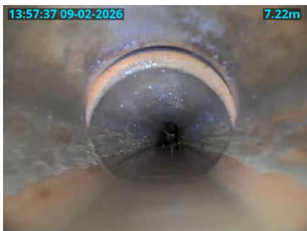
10BX_U_09022026_1357_021.jpg, 00:00:48, 7.22 m Joint displaced, medium
