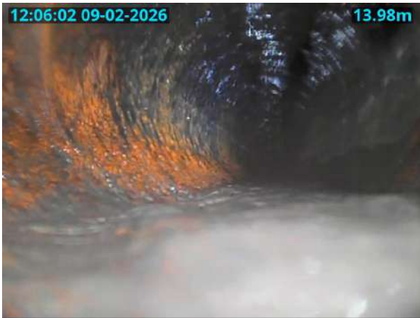
MH9X_D_09022026_1208_094.jpg, 00:01:49, 13.98 m General photograph taken at this point
