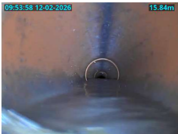
MH50X_5ff3765e-78a2-405e-8e3c-dcf9fef40dc9_20260223_123427_065.jpg, 00:01:52, 15.84 m Water level, 25% of the vertical dimension
