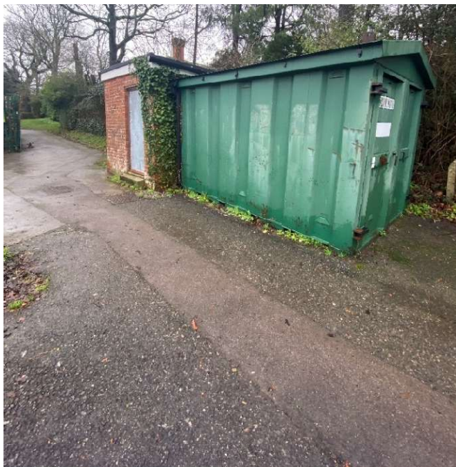
Existing hardstanding adjacent to building
