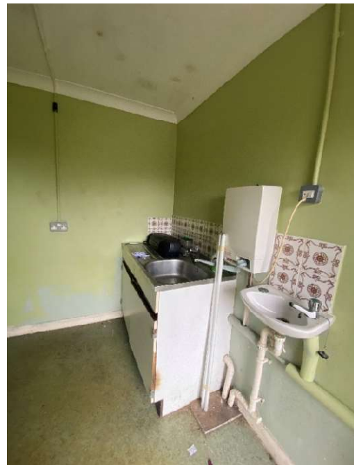
Interior view with existing sinks.
