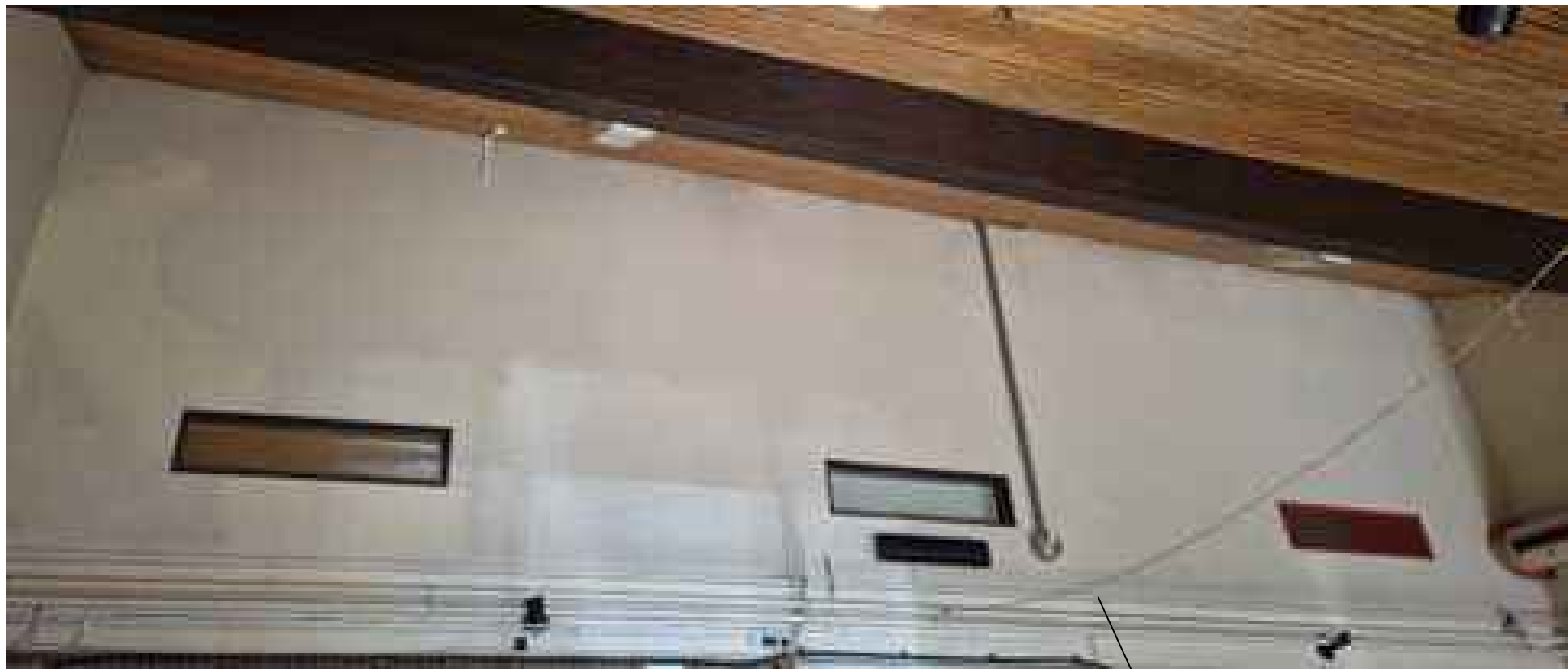
EXISTING VIEW OF AREA
