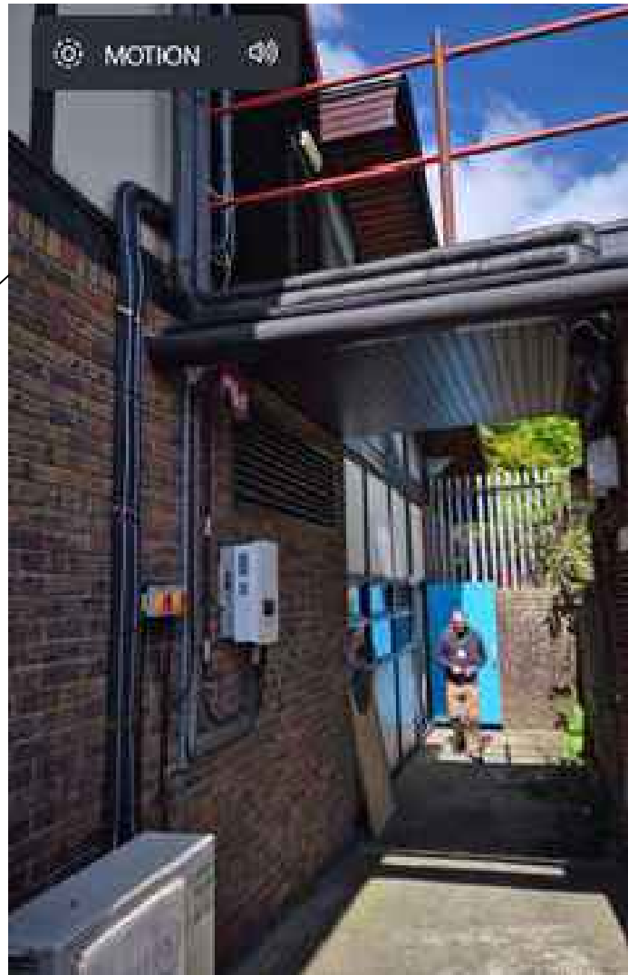
EXISTING VIEW OF AREA
