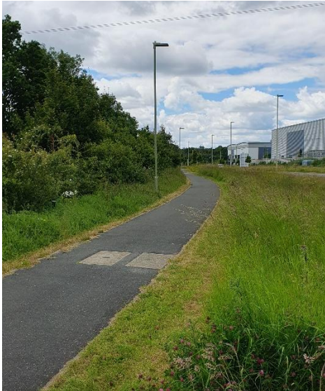
Photograph 4: Footway on southern side of Fitzwygram Way.
