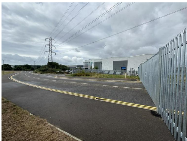
Photograph 1: Gated access to proposed Unit 400 location
