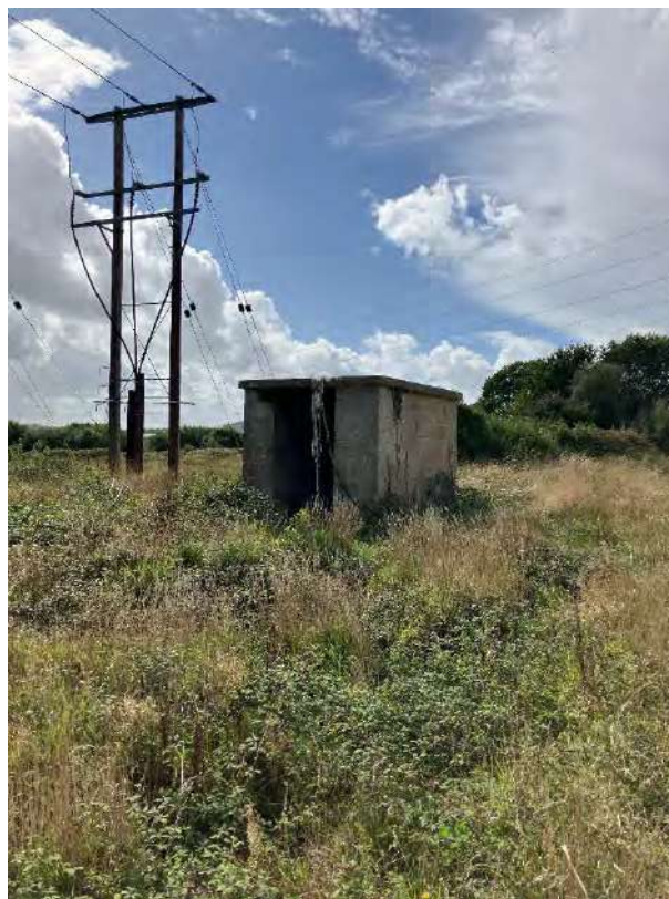
Figure 10: Small brick building in SE corner of site
