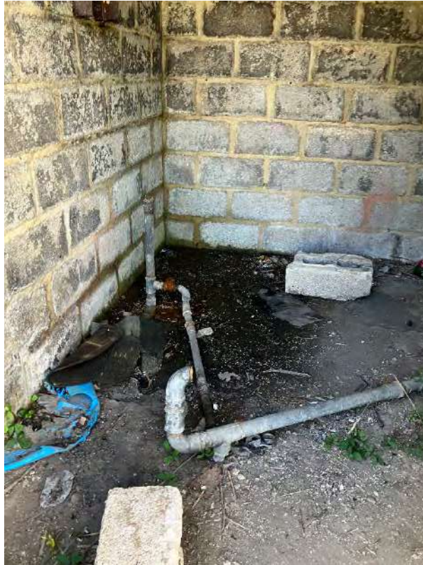
Figure 11: Inside brick structure
