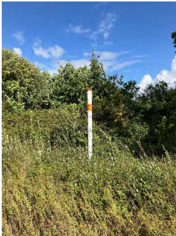
Figure 8: Gas main marker posts
