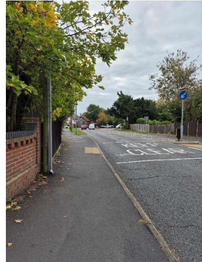
Photograph 80: Existing condition on Hulbert Road (B2150) towards Bedhampton Road
