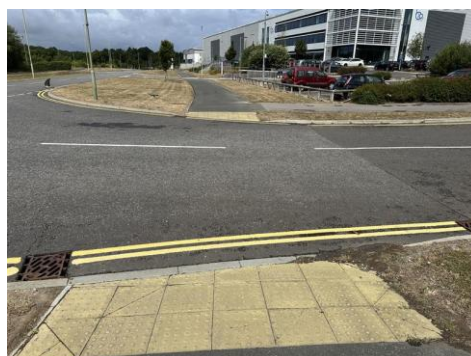
Photograph 14: Crossing Point across the access road to the north of Fitzwygram Road towards proposed site
