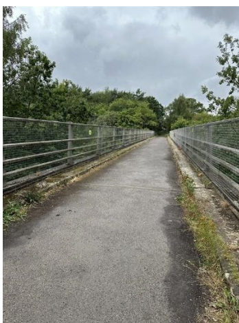
Photograph 35: Park Lane existing conditions heading over the bridge
