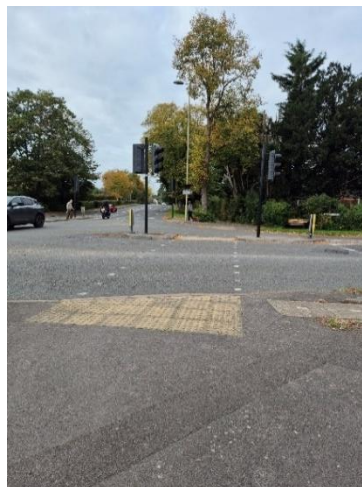
Photograph 81: Signalised crossing across Hulbert Road (B2150)
