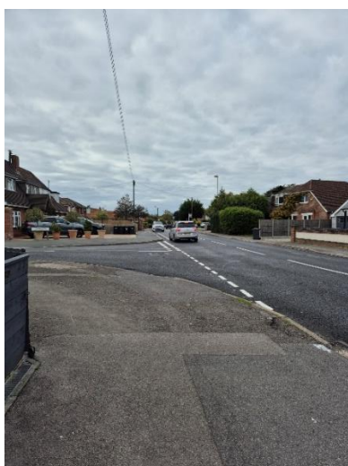
Photograph 77: Existing Conditions near Hooks Lane
