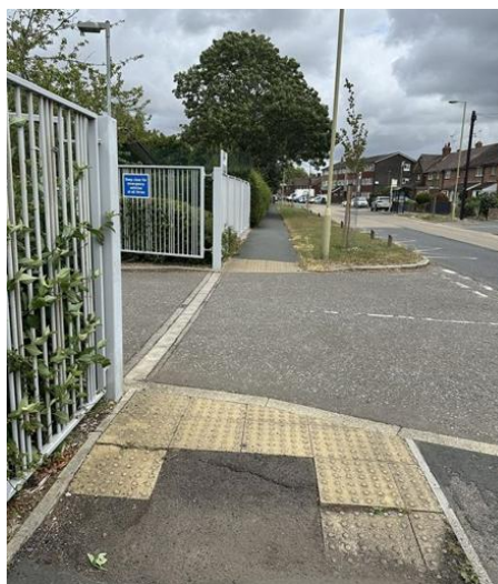
Photograph 63: Crossing point on Park House Farm Way across the Learning Centre entrance (looking north)
