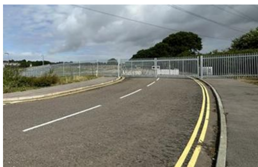
Photograph 7: Footways leading up to gated access
