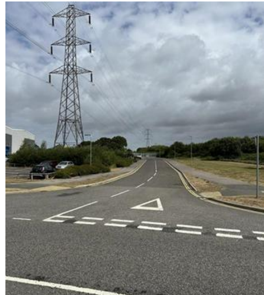
Photograph 10: Access Road off Fitzwygram Way towards Unit 400
