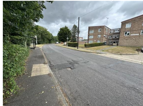
Photograph 27: Footway leading to the bus stop on Calshot Road & crossing point across carriageway (Southern edge of carriageway)
