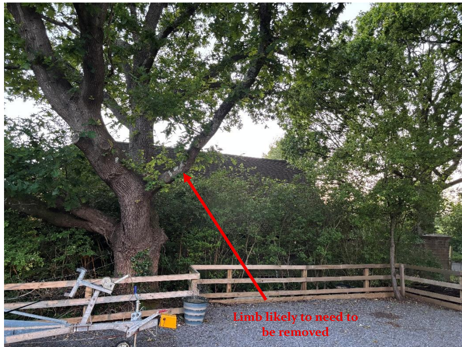
Photograph 1: Limb likely needing to be removed from tree T1 to allow car barn roof to be installed.
