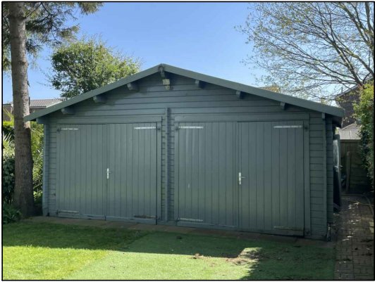
Existing garage (to be replaced)
