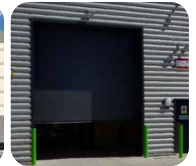
LOADING DOOR & STEEL BOLLARD
