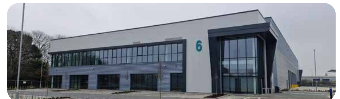
COMPLETED PHASE 2 DEVELOPEMT EXAMPLE
