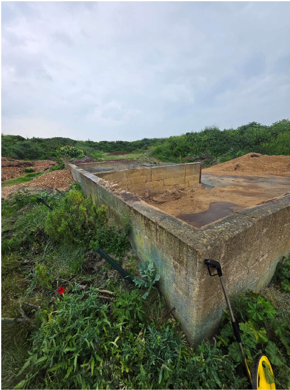
Figure 4 Area of tank location.
