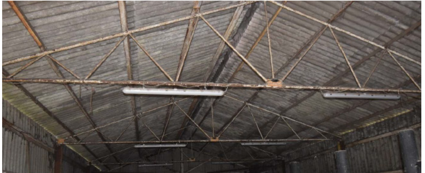
Steel Structural Frame
