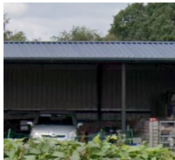
Nearby barn featuring metal roof
