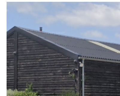
Nearby barn featuring metal roof and dark timber cladding
