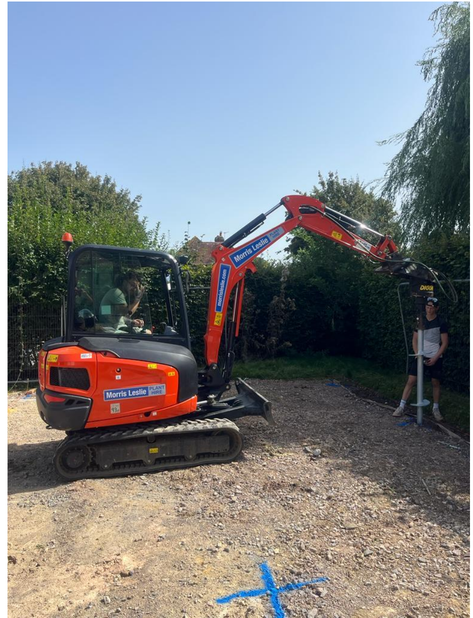
Preparing and inserting the screw piles at pre-set locations as marked out on the ground with blue crosses.
