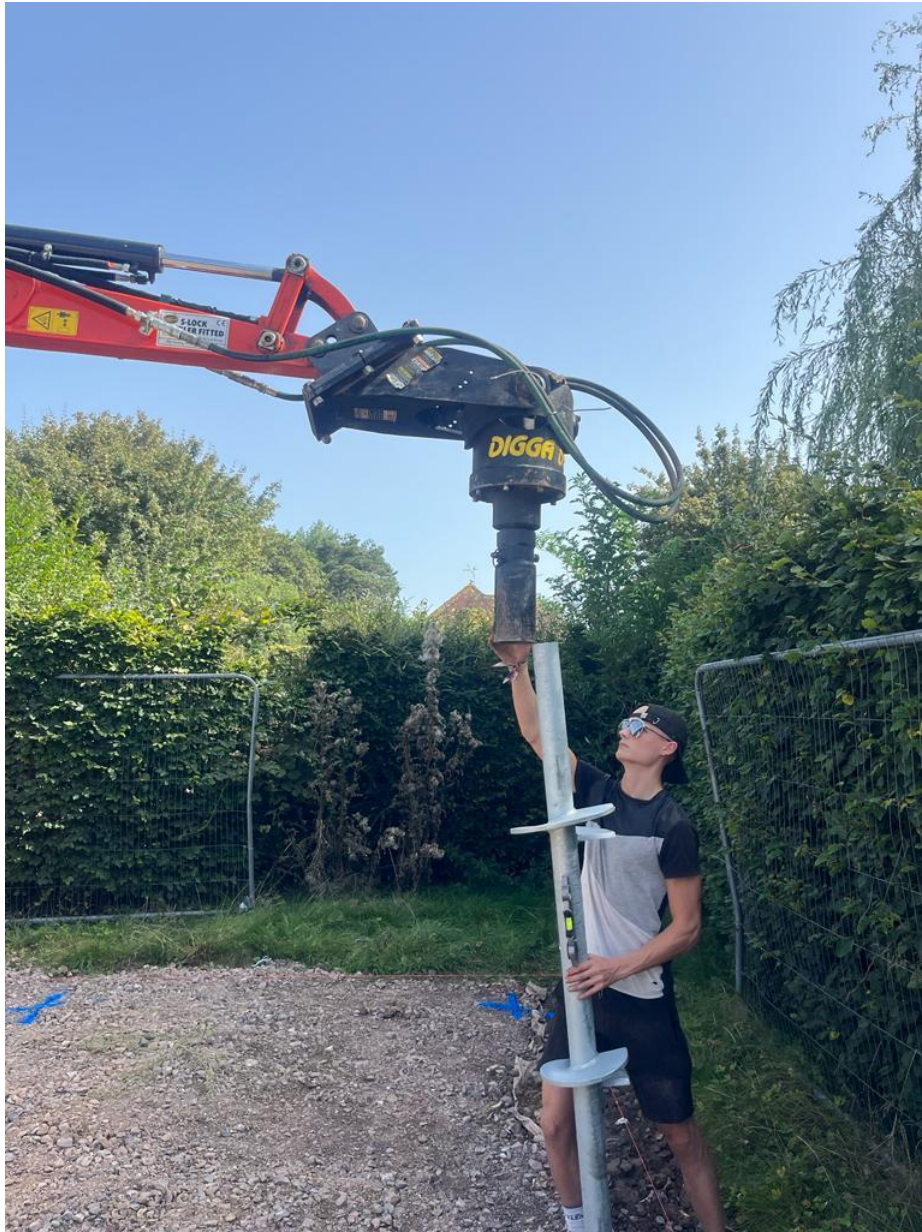
Preparing and inserting the screw piles at pre-set locations as marked out on the ground with blue crosses.
