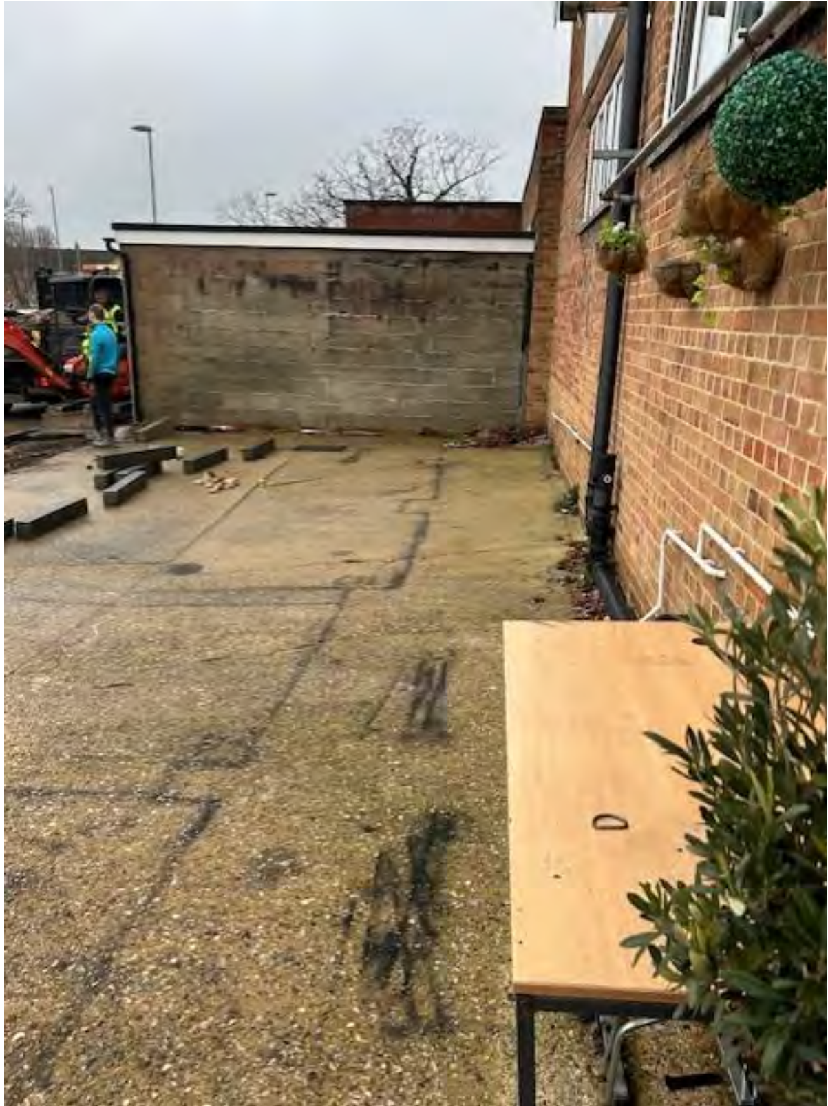
Photo 4: Downpipe and drainage pipe noted on the exterior of the building
