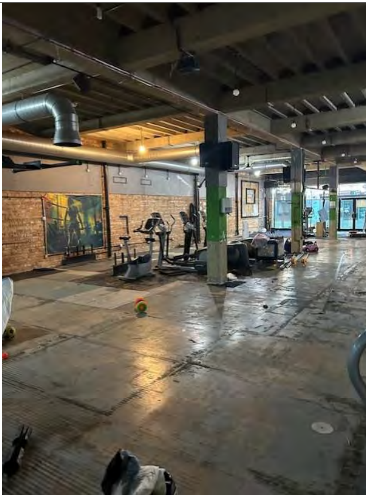
Photo 2: Hardstanding ground flooring inside the building
