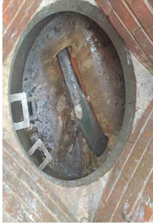
Manhole Open Photo:
