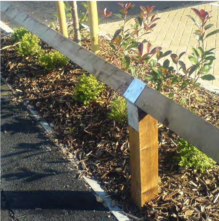
Knee rail fencing (Birdsmouth fencing)
