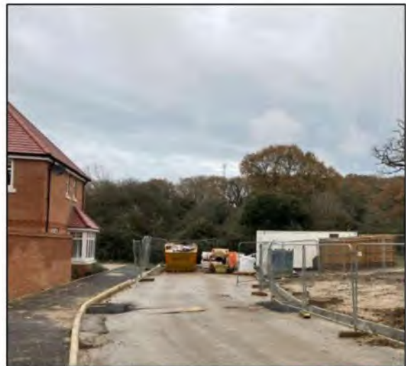
Photograph 3: End of Road at Wilkes Way
