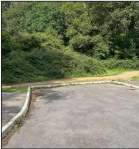
Photograph 2: End of Road at Merritt Way
