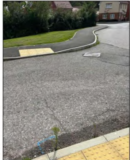
Photograph 9: Crossing Point across Baker Close
