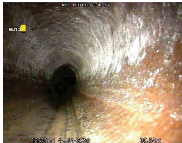
4, 00:03:34, 30.54 m Finish connection without manhole, Down Line, the pipe is flowing fine
