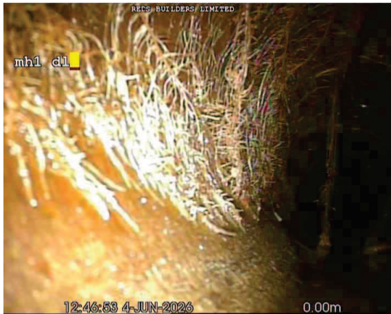
1, 00:00:00, 0.00 m Start manhole, Mh1
