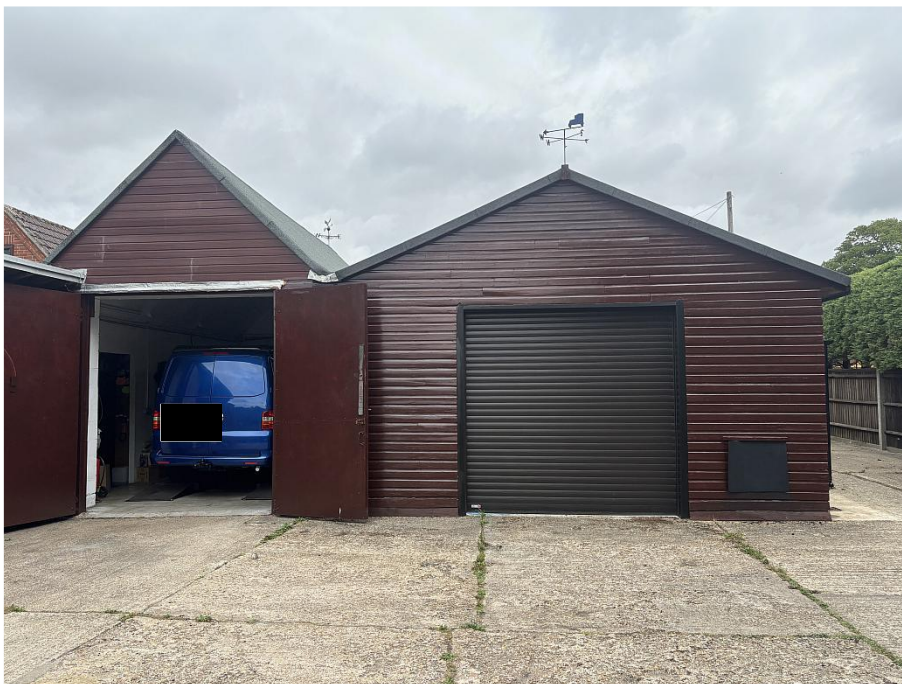
Timber workshop extensions to the rear of the original brick garage
