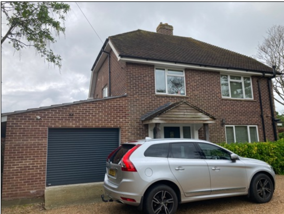
Photograph 2. Northern and elevation of residential property (Jacaranda).
