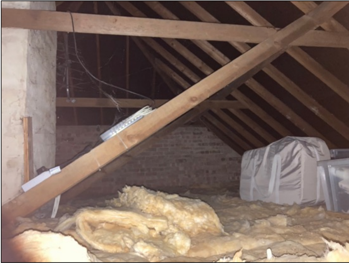
Photograph 3. Internal loft space.
