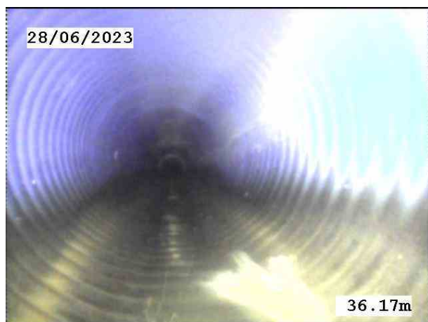
SW04X_1a7e42ed-a6e0-4eac-acbc-5fe197bd6c0f_20230628_103225_288.jpg, 00:02:40, 36.17 m Pipe material changes to polyethylene at this point
