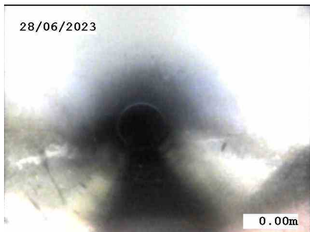
SW04X_6a7cd6eb-fe49-4839-b4e5-7ce88a73c9d5_20230628_102910_199.jpg, 00:00:01, 0.00 m Start node, manhole, reference: SW04
