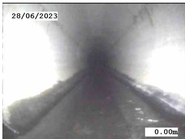
SW01X_eac7cad6-82ca-4c64-a27b-fb695524fdcd_20230628_090816_977.jpg, 00:00:01, 0.00 m Start node, manhole, reference: SW01
