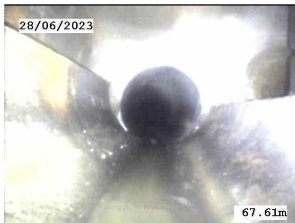
SW04X_b087a2c8-f755-4acb-929d-ddb4a17bd0cd_20230628_103606_940.jpg, 00:06:15, 67.61 m Finish node, manhole, reference: X, SW05
