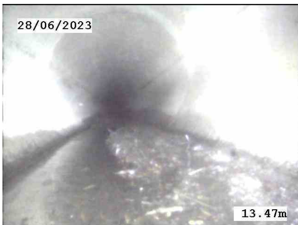
SW02X_11b0ae67-455b-44dd-81f4-62b310ac079b_20230628_092248_052.jpg, 00:01:07, 13.47 m General photograph taken at this point
