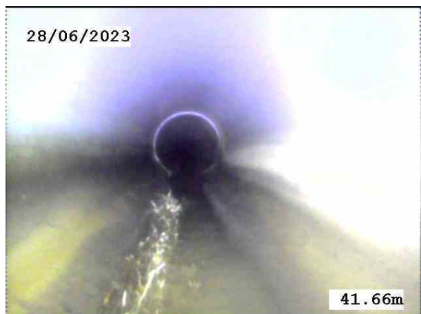
SW04X_048cf9ac-950e-4cea-84f7-15bdcdfc2dcb_20230628_103332_741.jpg, 00:03:54, 41.66 m Pipe material changes to vitrified clay at this point
