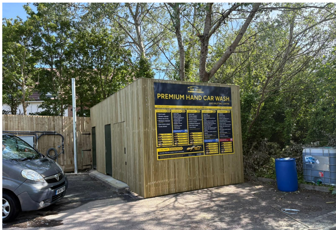
Figure 6 – As Built Storage Unit/Office with new timber façade treatment
