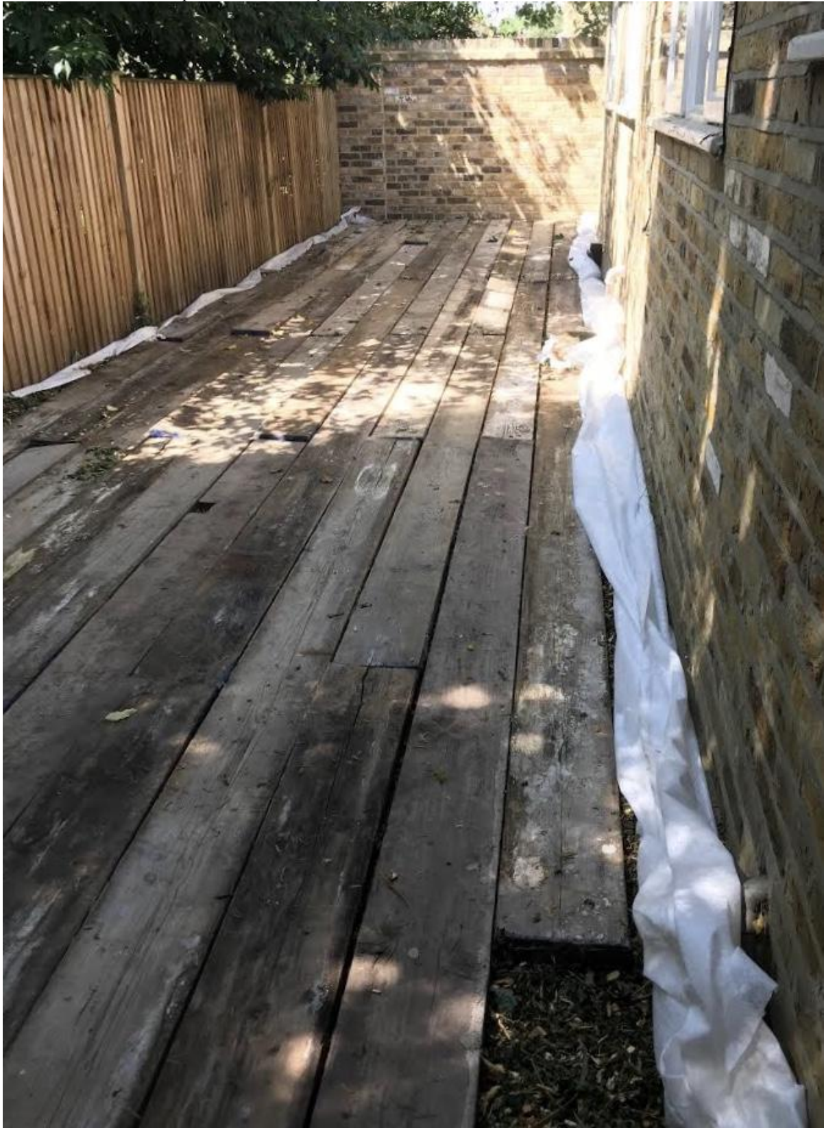
Photo 1. Scaffold boards placed on woodchip
