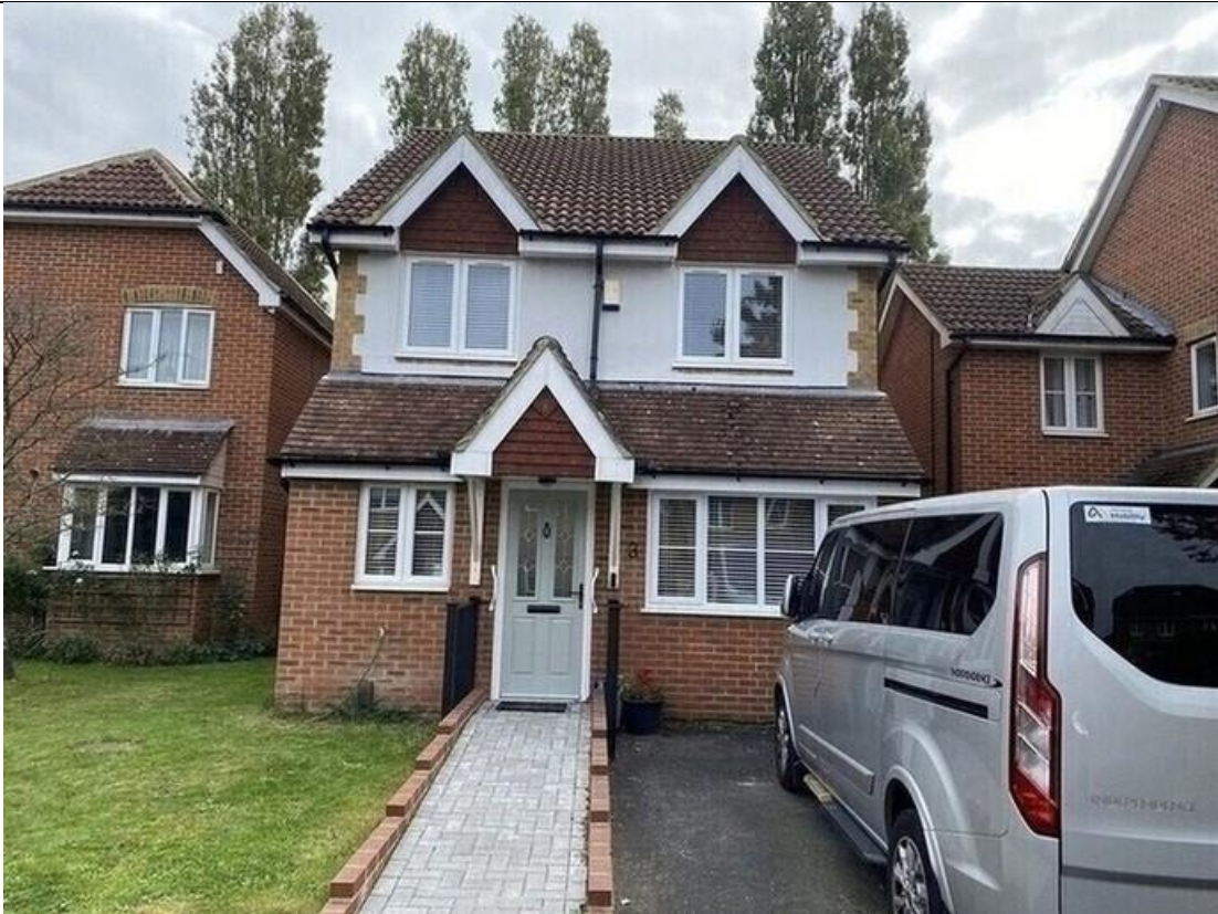
Front Elevation of Risk Address
