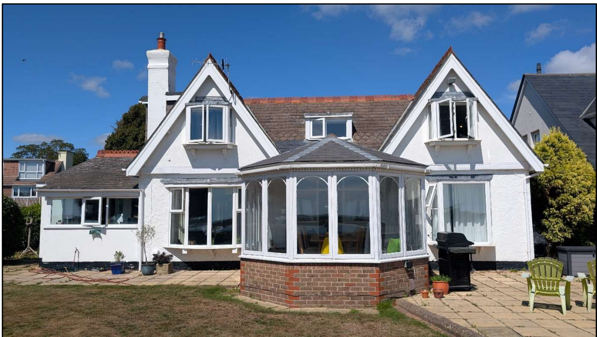
Photo 2 – View of B1 from the south.
