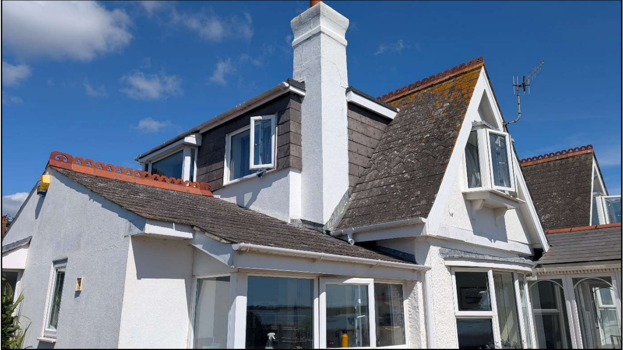
Photo 3 – View of the complex roof.
