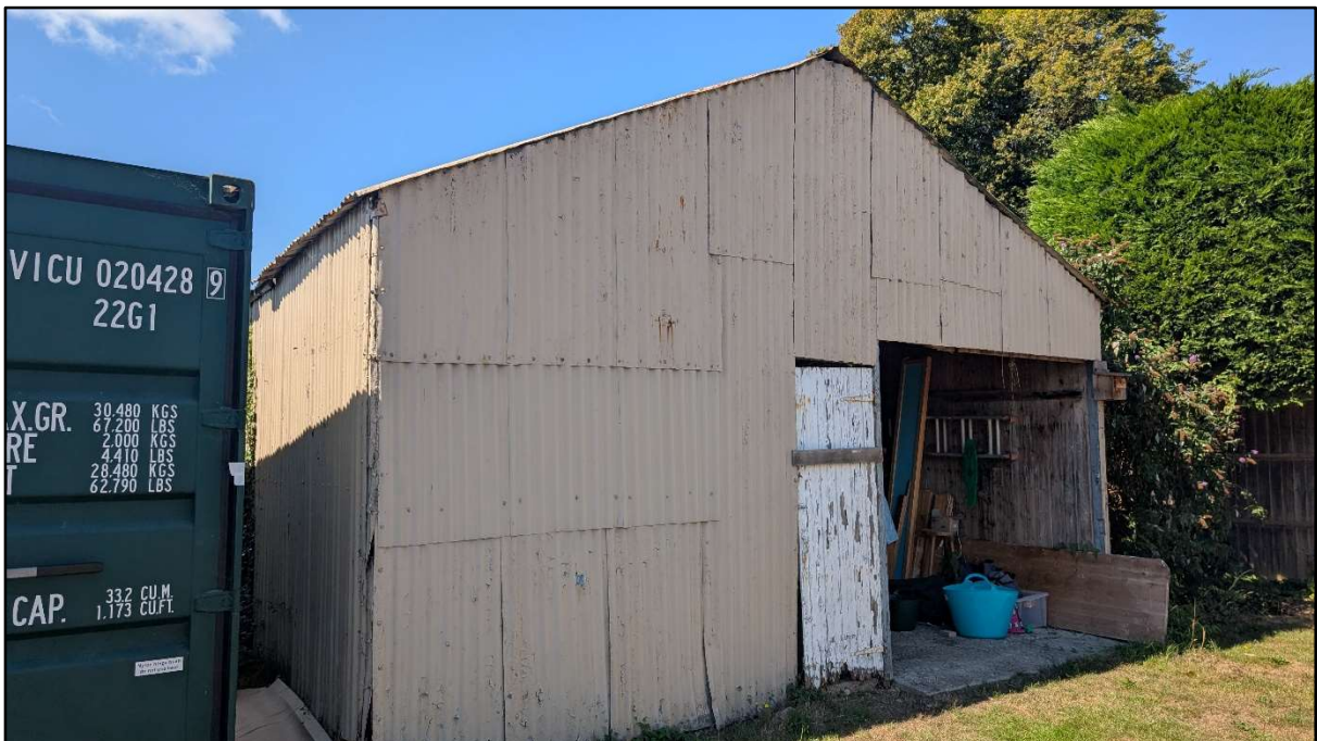
Photo 8 – View of B2 from the east.
