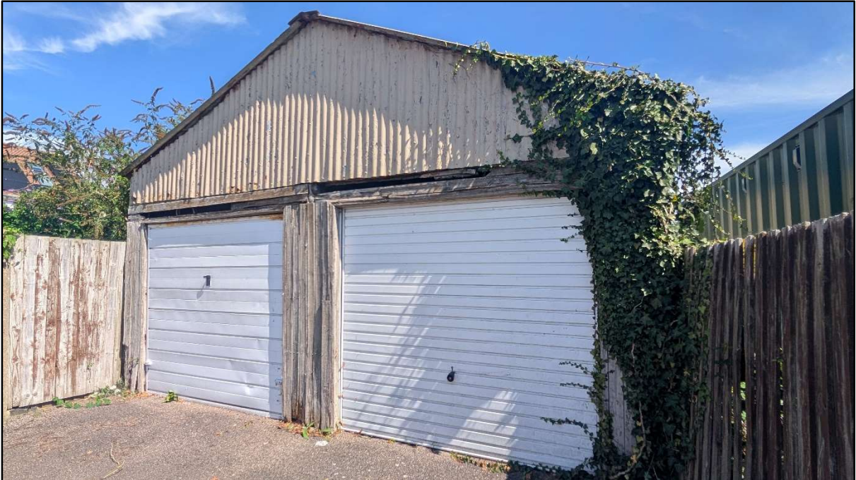
Photo 7 – View of B2 from the west.
