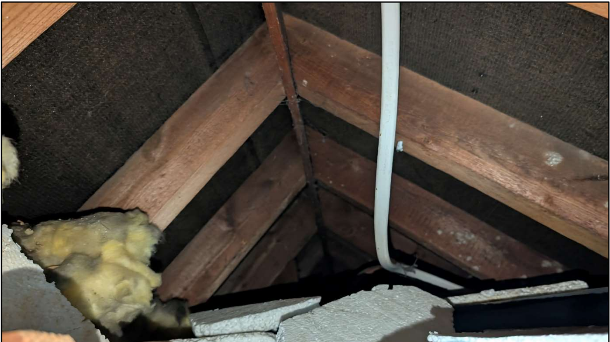
Photo 6 – View inside the loft void in B1.
