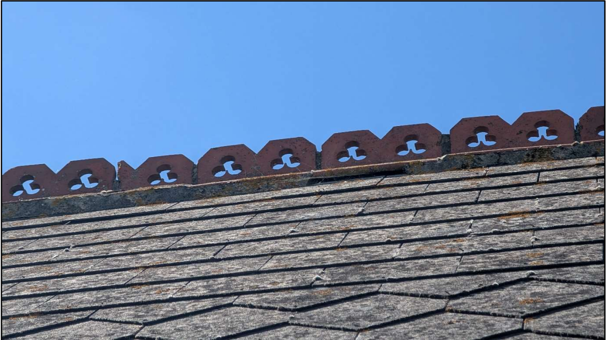
Photo 5 – View of the ornate ridge tiles to be removed carefully as a matter of course.
