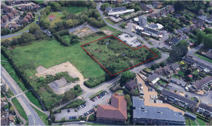
Aerial view from the northwest.
