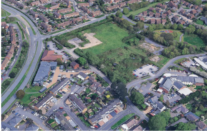
PHOTO 1: Aerial view of the site from the southwest.
