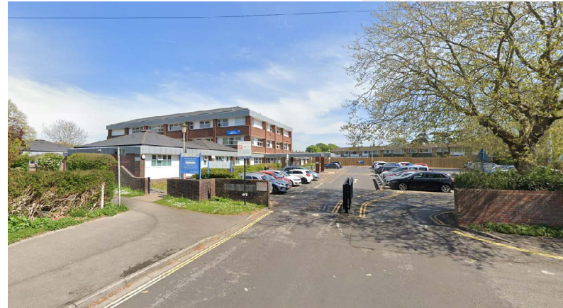
PHOTO 5: Nearby Havant Health Centre.
