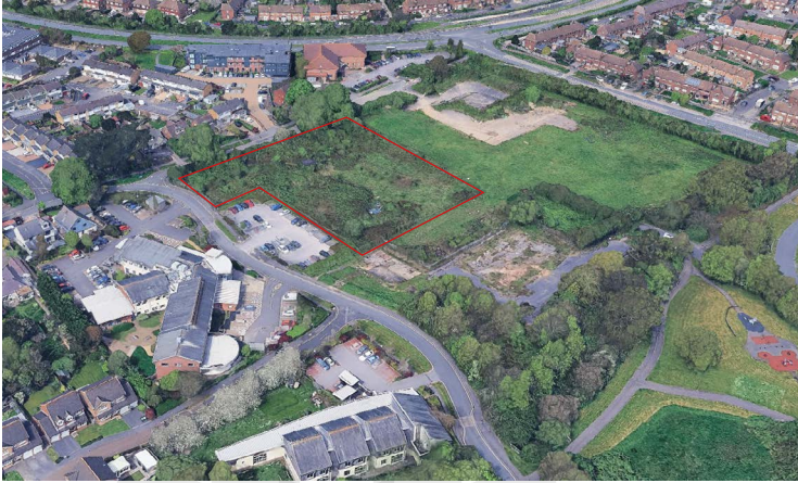
Aerial view from the southeast.
