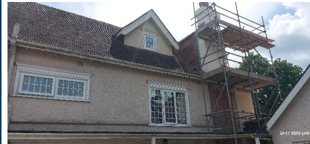
Photo 3: South facing pitched roof with clay tiles
