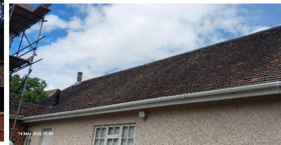
Photo 3: South facing pitched roof with clay tiles
