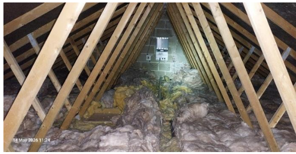
Photo 15: Outhouse loft void
