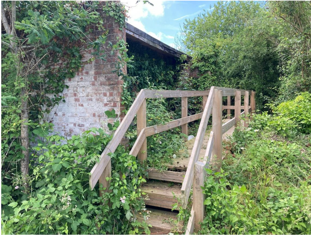
Wooden bridge providing access to the site
